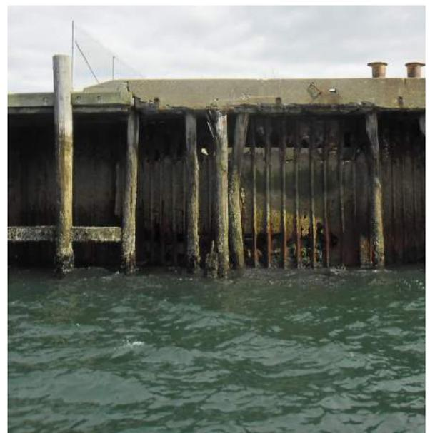
Damage to the South and East Jetties has reduced their structural capacity.
