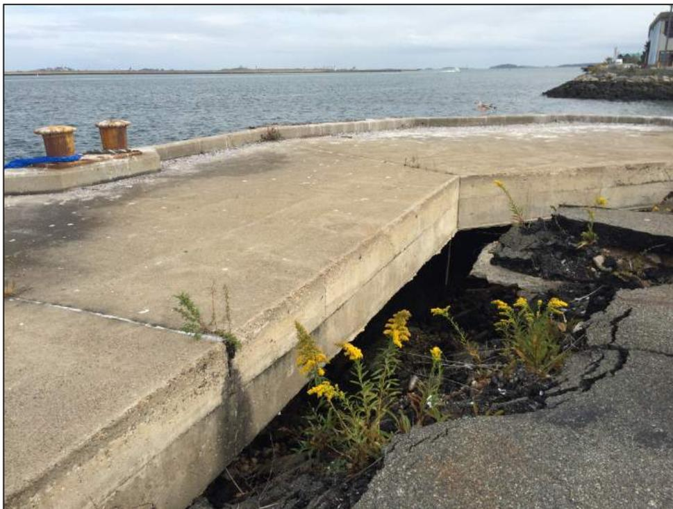
Figure 16: View of open sinkhole in the deck of Dry Dock #4.
