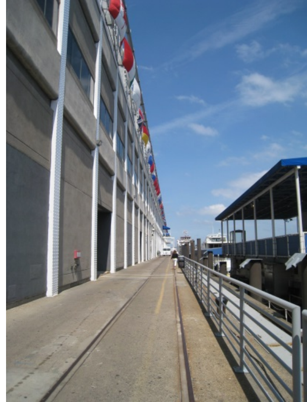
East façade & apron / Harborwalk
