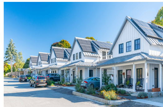
BUILDING PRECEDENT DESIGN EXAMPLE. NOTE THE BAT AND BOARD SIDING WITH METAL ROOFING AND BLACK WINDOW FINISHES.
