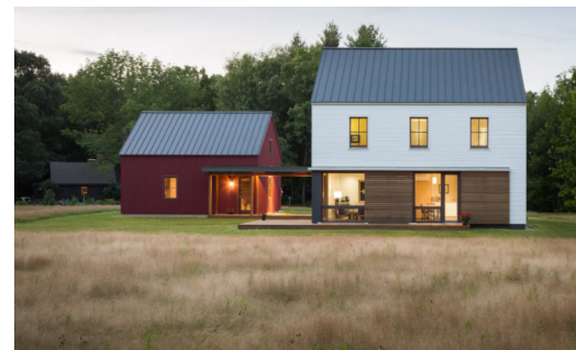
BUILDING PRECEDENT DESIGN EXAMPLE. NOTE THE CHANGE IN MATERIALS AT ENTRANCES BUT SIMPLE BARN STYLE DESIGN.
