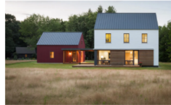
BUILDING PRECEDENT DESIGN EXAMPLE. NOTE THE CHANGE IN MATERIALS AT ENTRANCES BUT SIMPLE BARN STYLE DESIGN.
