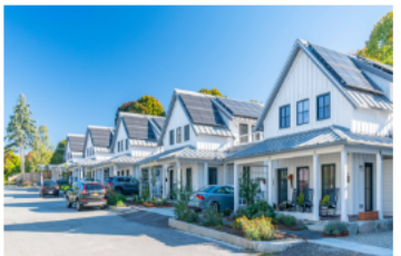
BUILDING PRECEDENT DESIGN EXAMPLE. NOTE THE BAT AND BOARD SIDING WITH METAL ROOFING AND BLACK WINDOW FINISHES.
