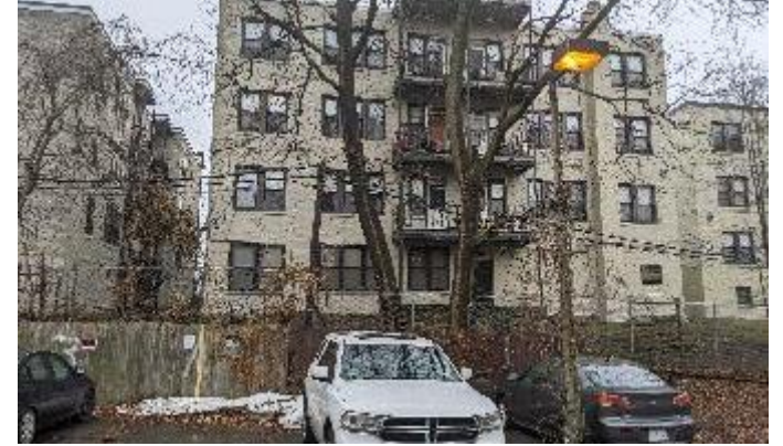
Apartment Property Building SQFT: 21,168 Owner: 182 Park Gardens Association
