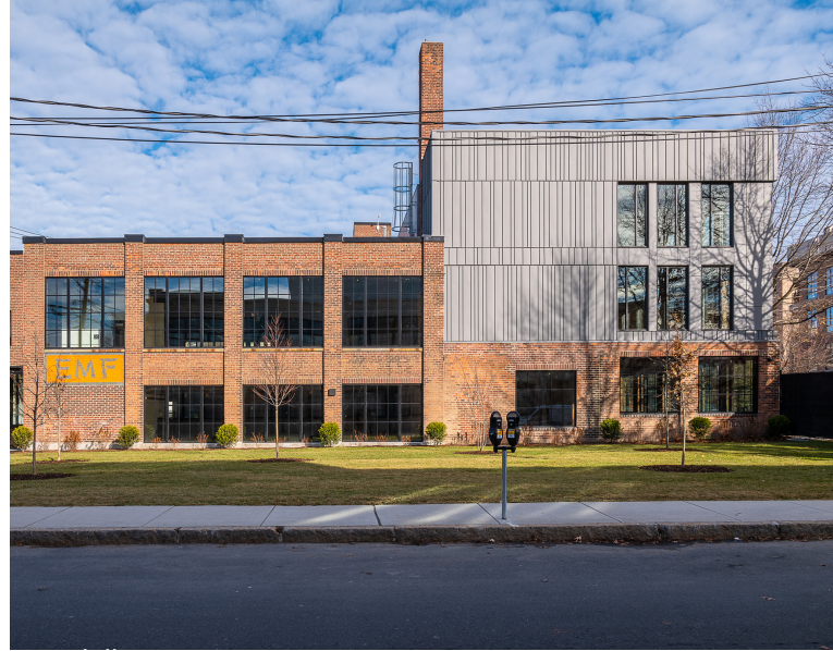
Seamed Metal Facade
