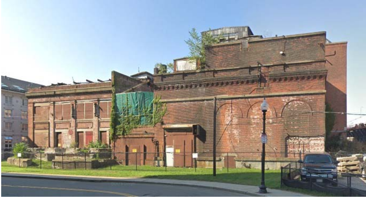
Figure 1-Building 108 Photo from RFP
