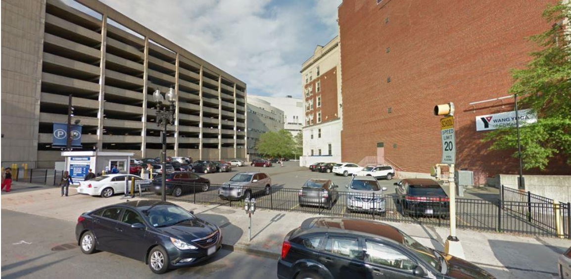
Existing Conditions at the Property.
