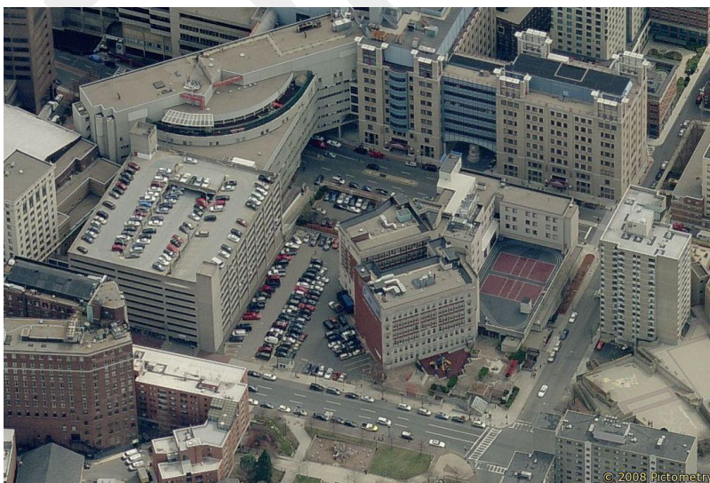
Aerial View of the Property.
