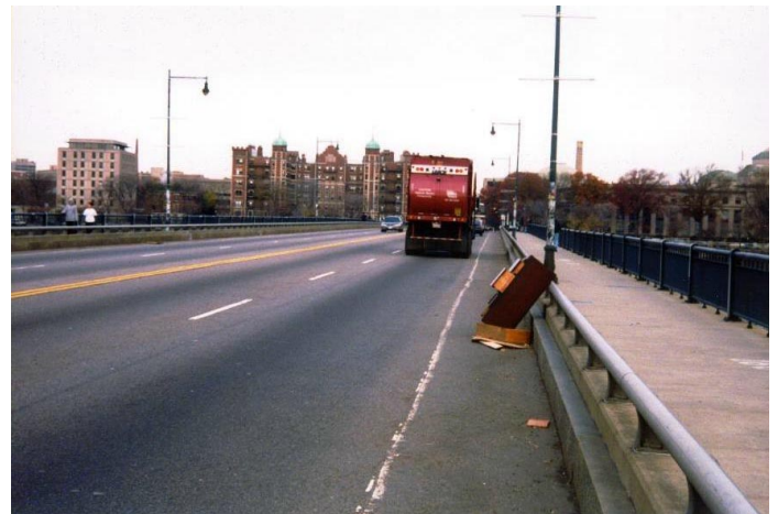
Repairs to this section of failed pavement and removal of debris from this roadway shoulder will improve bicycling conditions on these bridges.
