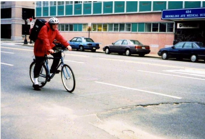
Roadway maintenance is important for the safety of bicyclists. Hitting a pothole can cause a serious fall or result in a crash with a motor vehicle.
