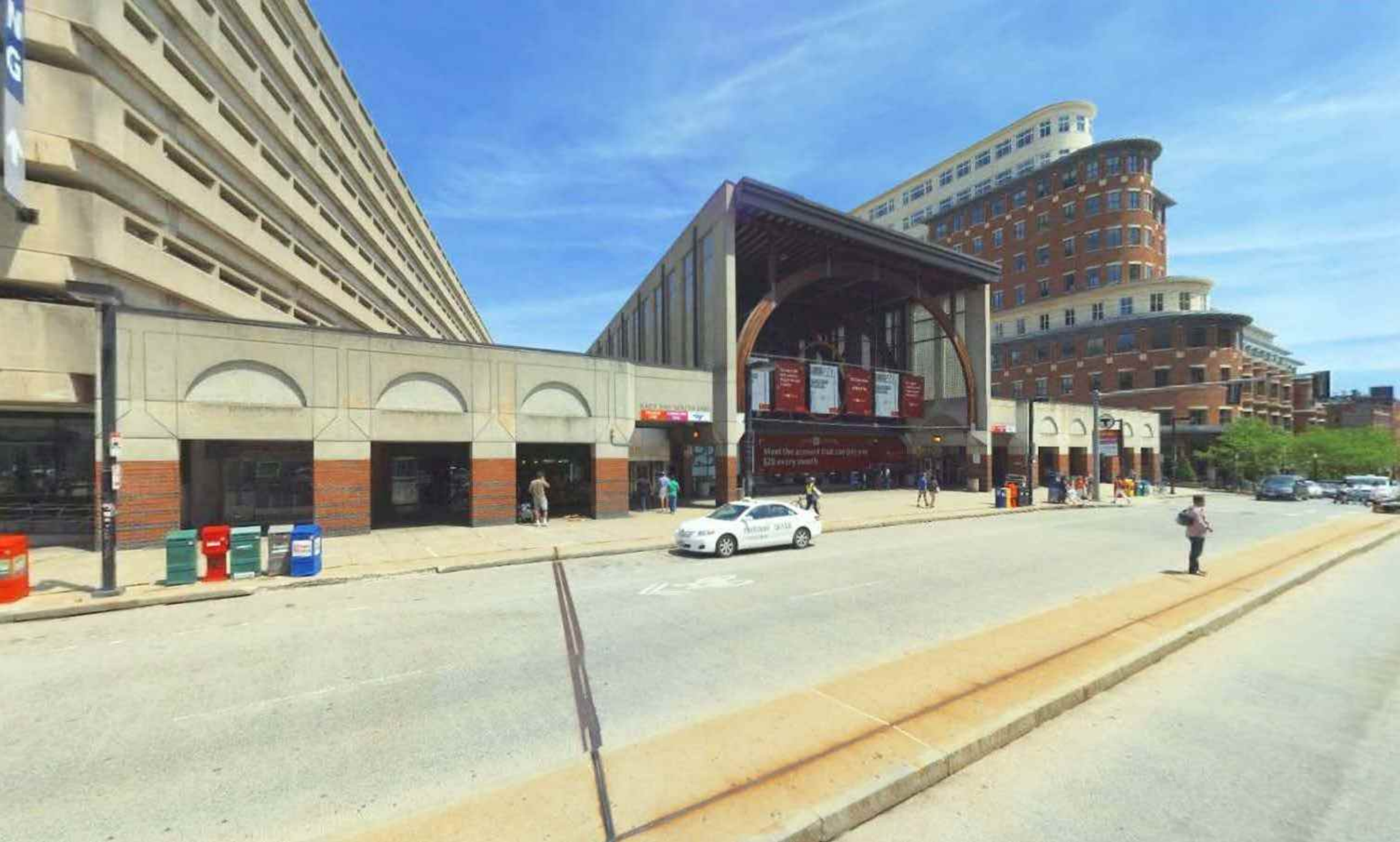
VIEW FROM DARTMOUTH STREET - EXISTING CONDITION
