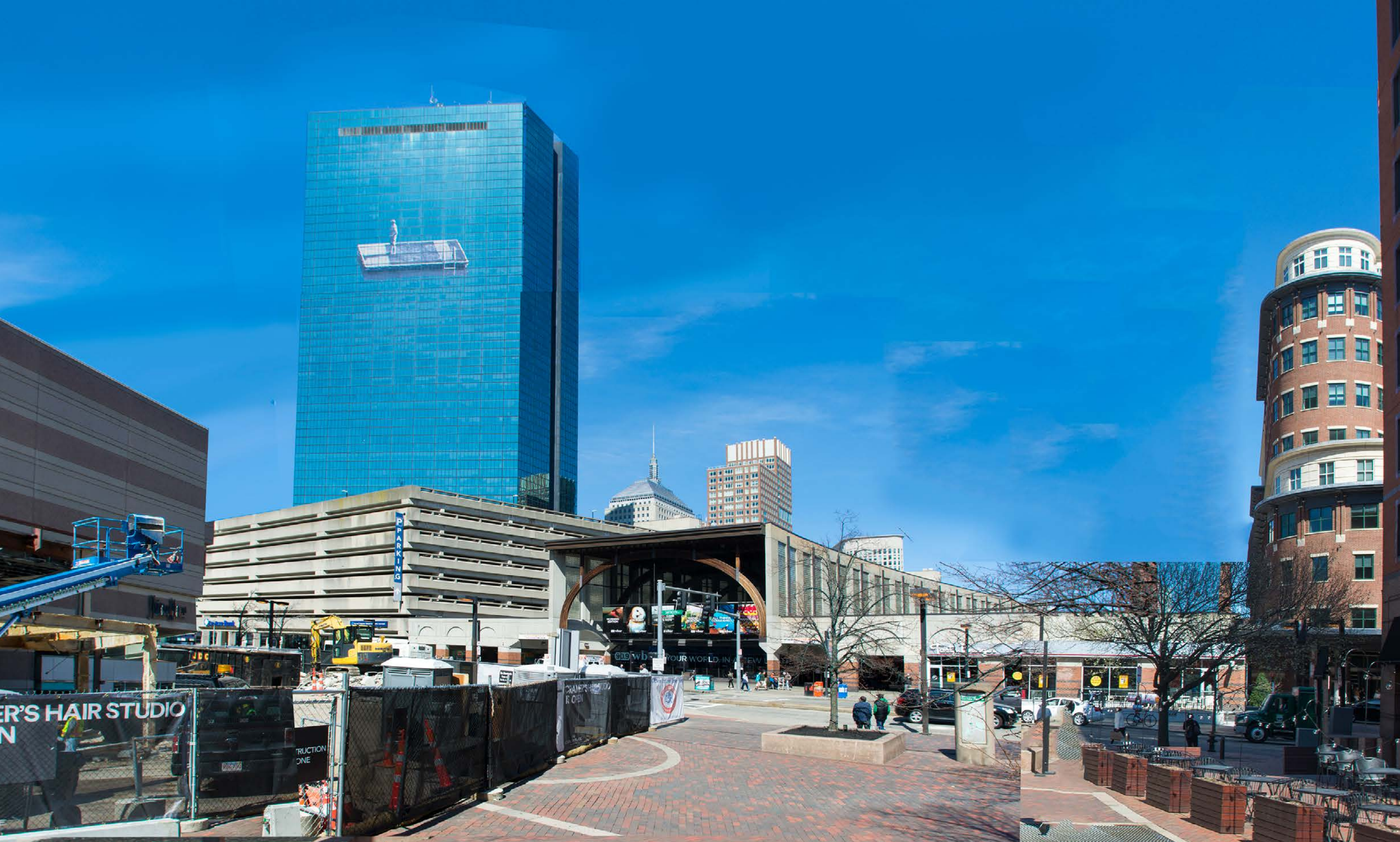
VIEW FROM SOUTHWEST CORRIDOR - EXISTING CONDITIONS
