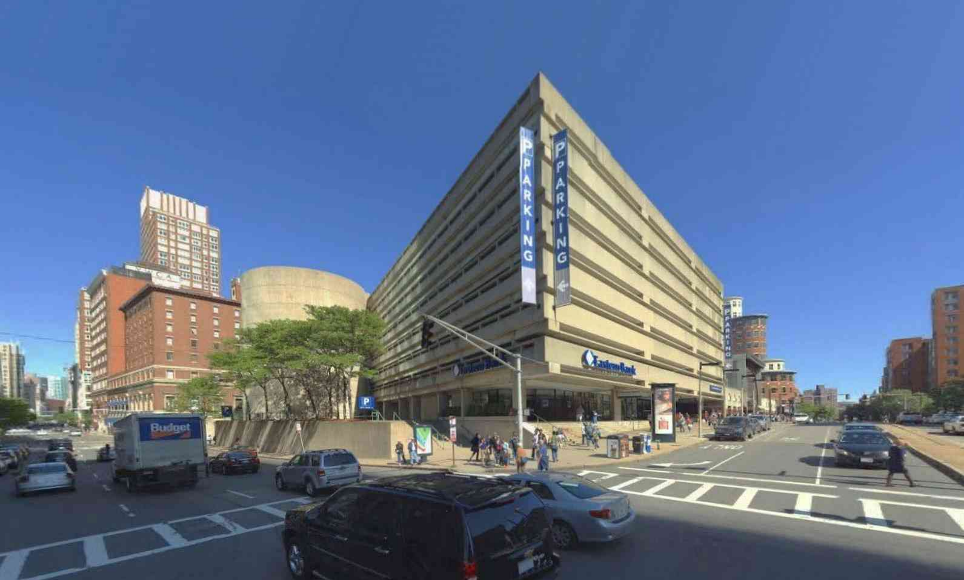
VIEW FROM DARTMOUTH STREET AND STUART STREET - EXISTING CONDITION
