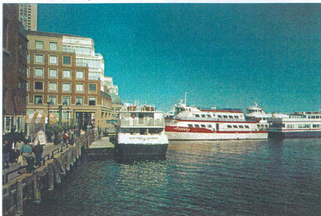
Rowes Wharf/400 Atlantic Avenue Terminal - Existing Conditions
