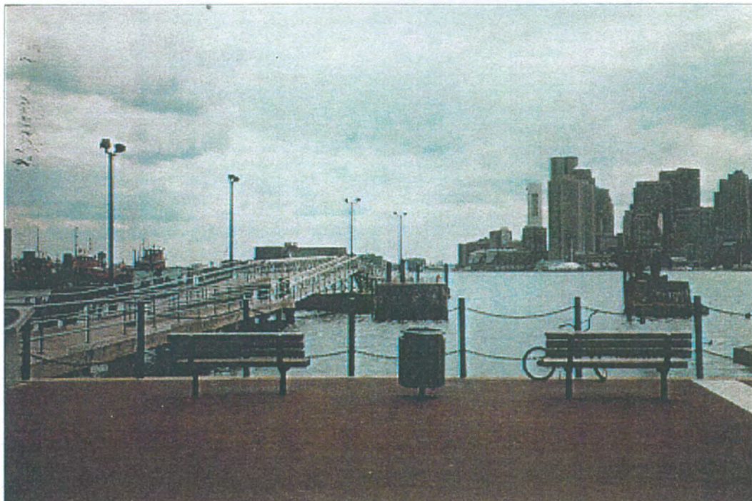
Lewis Mall Terminal, East Boston
