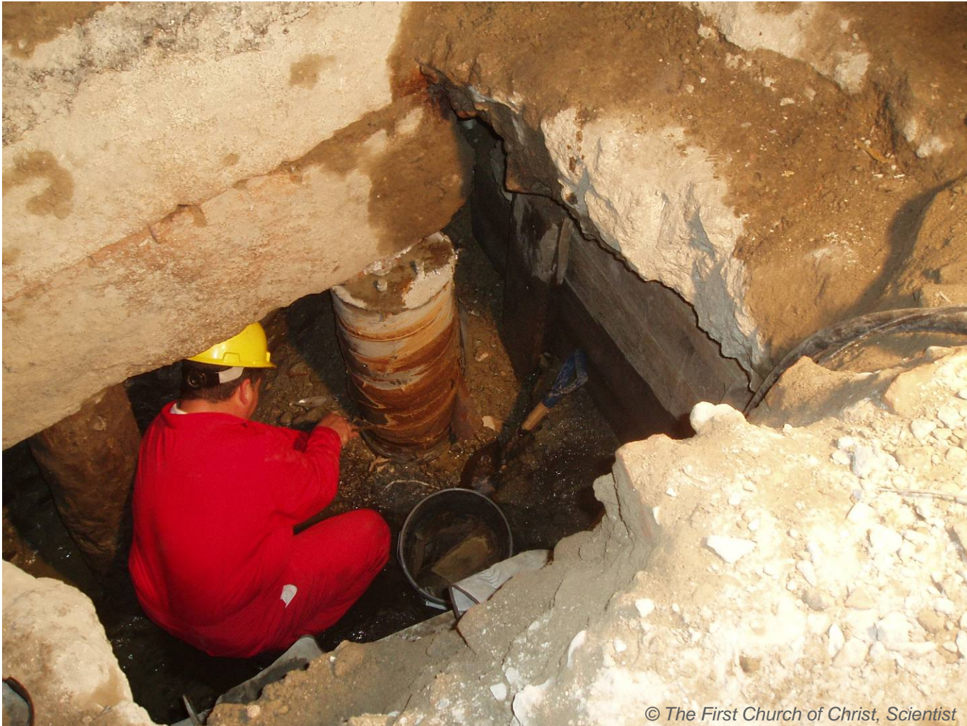
Surveying Pile Condition
