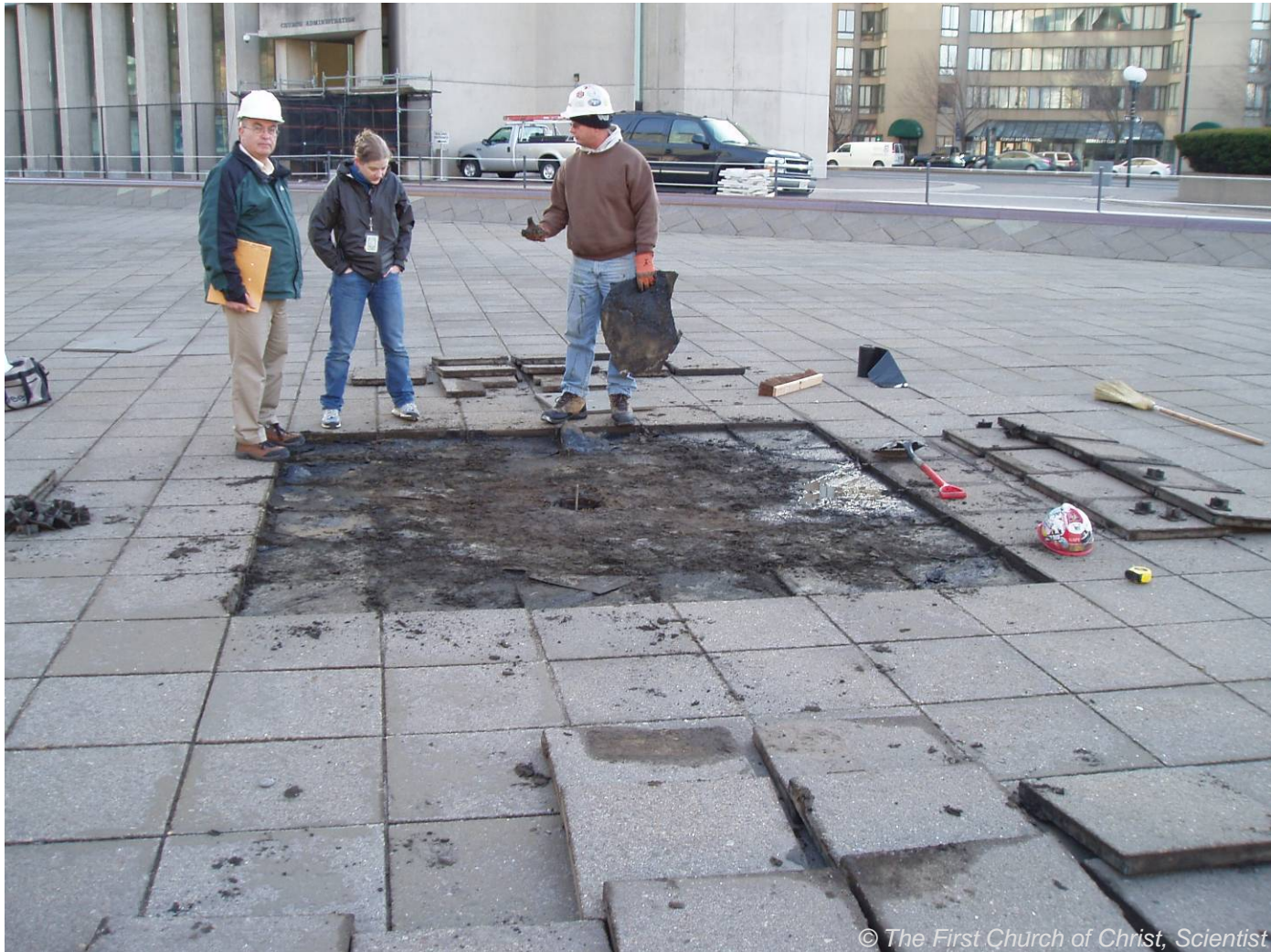
Surveying Waterproofing Membrane in Reflecting Pool
