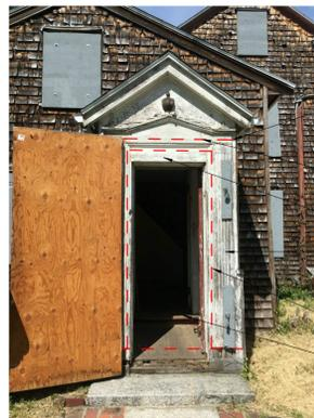
EXISTING DOOR AND ENTRY VESTIBULE IS NOT ACCESSIBLE AND MUST BE MODIFIED. EXTERIOR GRADE WILL BE RAISED 11" TO MEET NEW DOOR THRESHOLD HEIGHT WHICH WILL ALIGN WITH NEW FINISH FLOOR. DOOR WILL WIDEN TO ALLOW FOR 32" CLEAR OPENING. TRIM WILL BE MODIFIED TO ACCOMMODATE THESE CHANGES.
