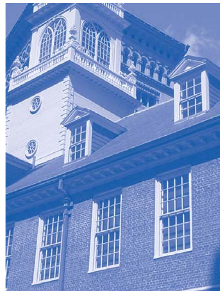
The Old State House (c 1713) is one of several historic sites on Boston's Freedom Trail, which winds through Downtown Crossing.
