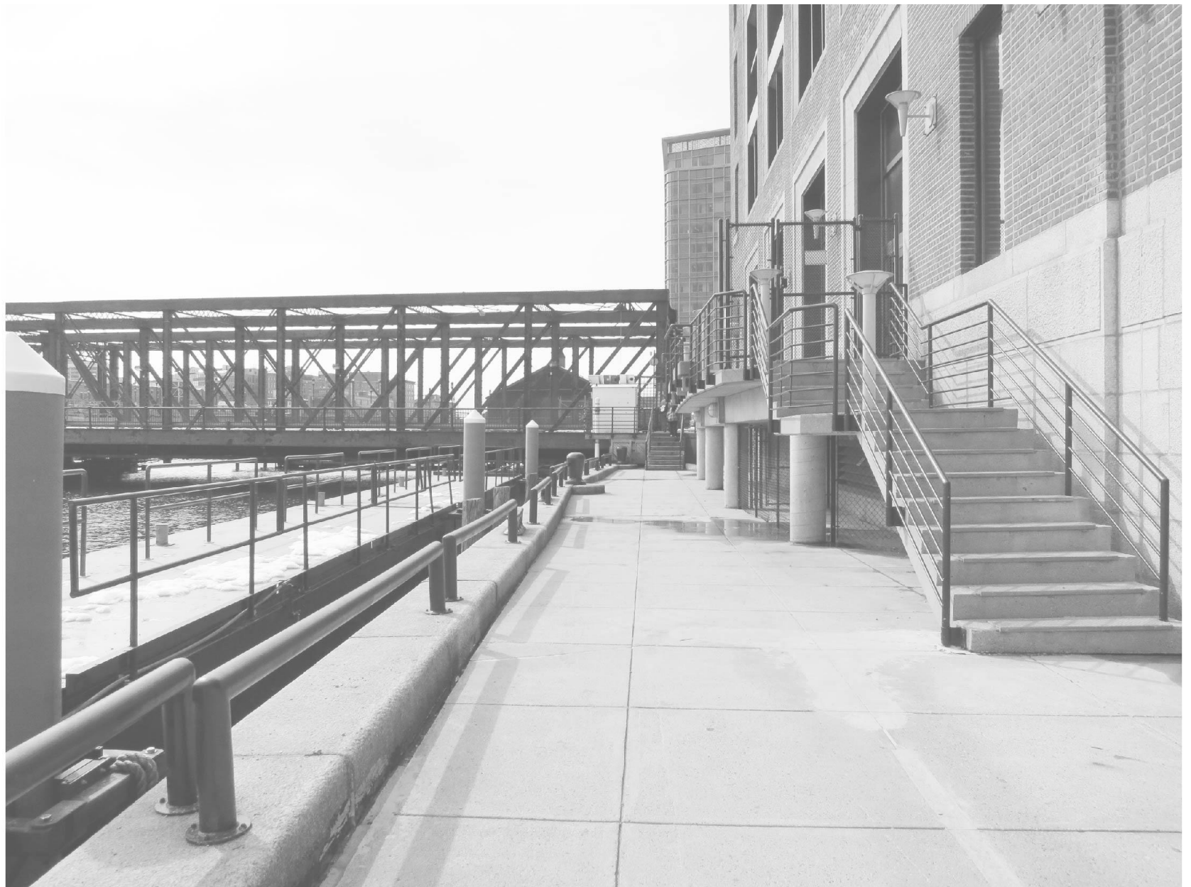
Northern Avenue Bridge / Hook
