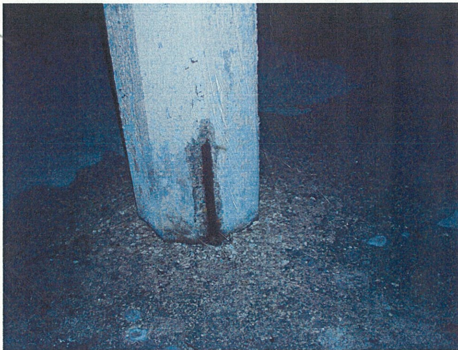
Photo CT0.6 – 5 th Floor Column Location of column where sample was taken.
