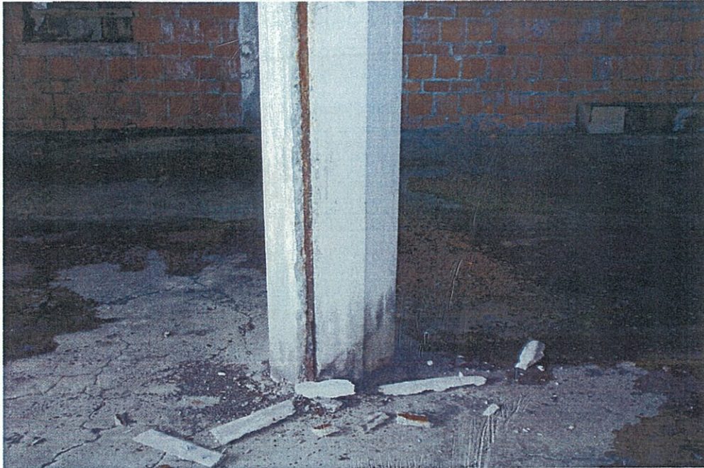
Photo G2.3 – 2 nd (Mezzanine) Floor
