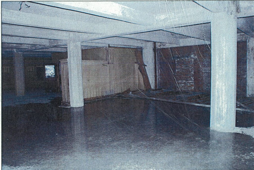
Photograph 14. Interior, , typical structure and layout of slab, columns, and beams.
