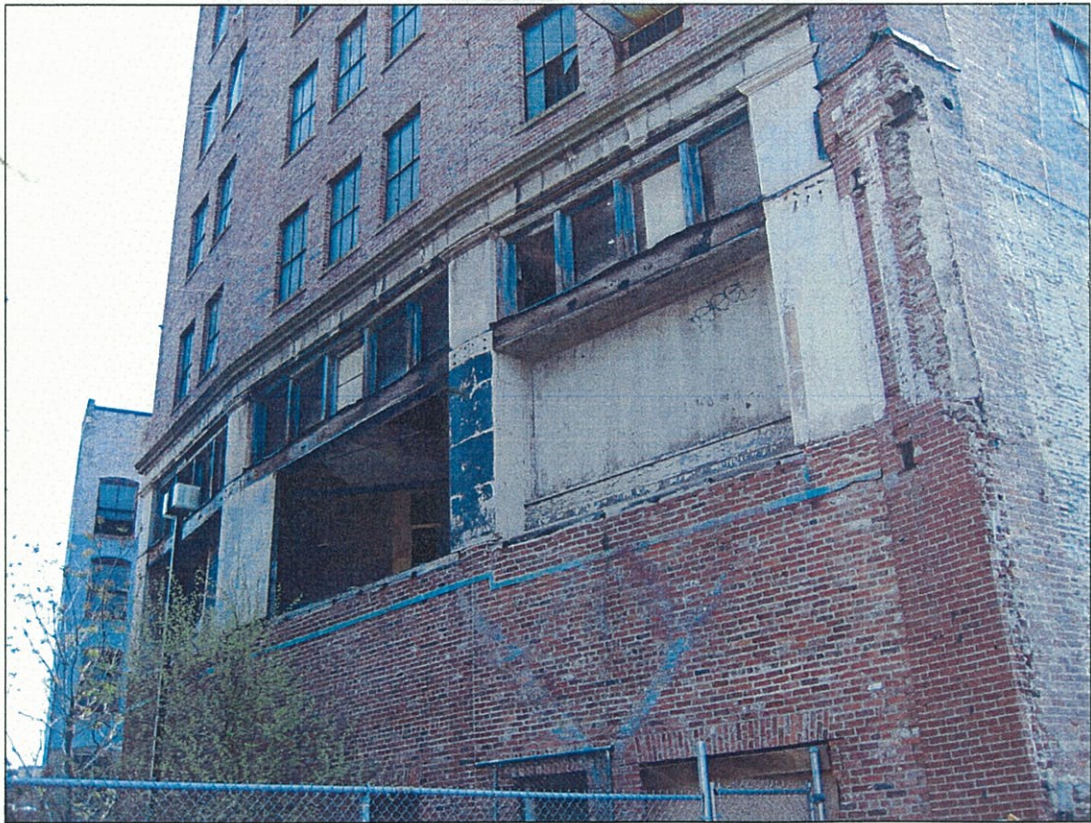
Photograph 8. Side and rear elevations detail, view northeast.
