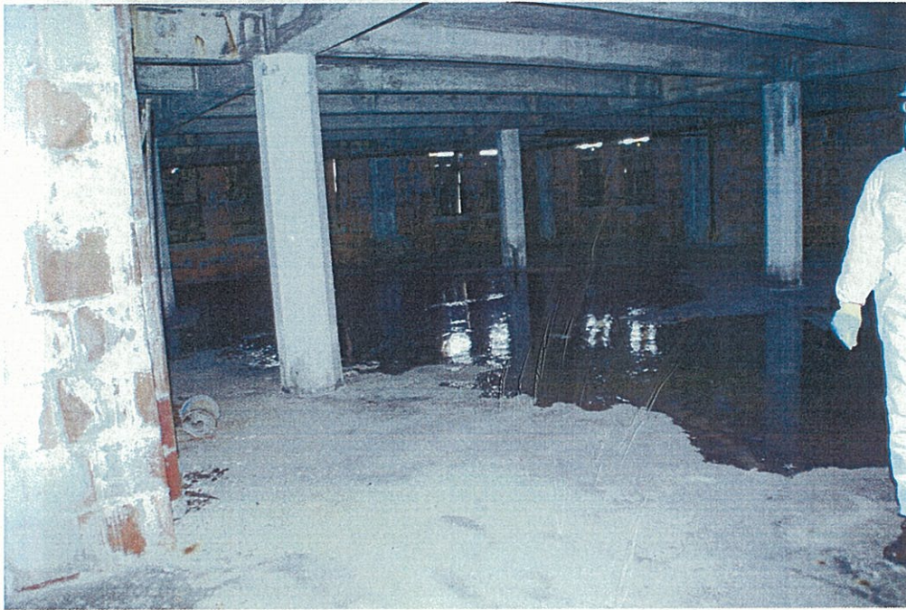
Photo G6.3 – 6 th Floor
