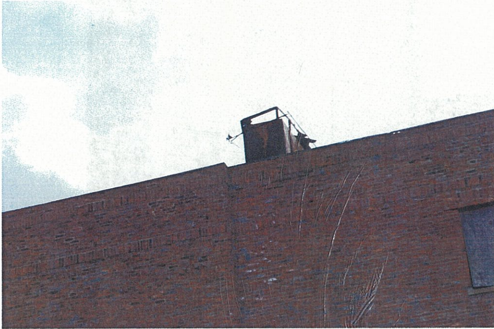
Photo GEX.7 – Partial Elevation Some rooftop equipment seen, not inspected.
