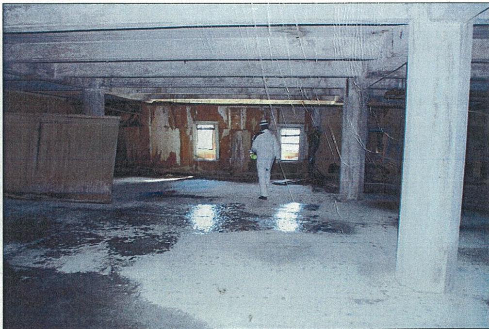
Photograph 16. Interior, typical structure and layout of slab, columns, and beams.
