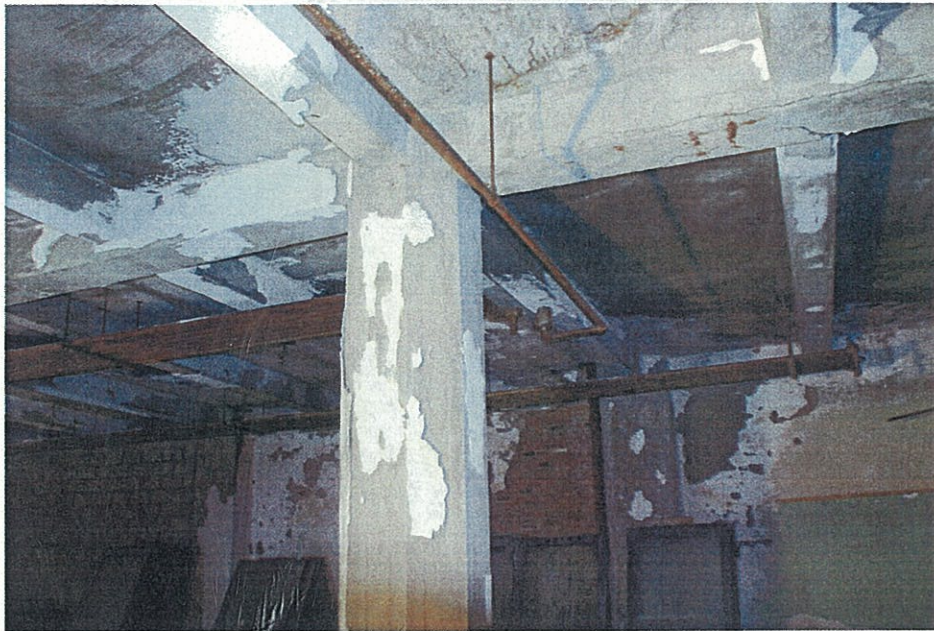
Photo G0.5 - Basement Typical beam-to-column framing.
