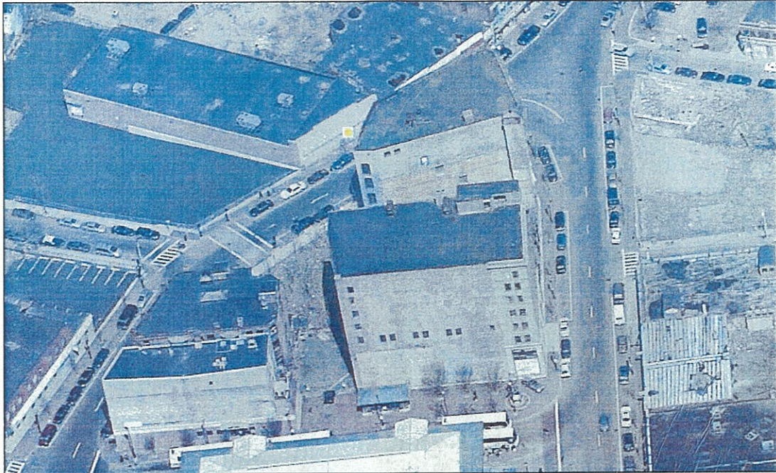
Photograph 1. Aerial view of site, view north.
