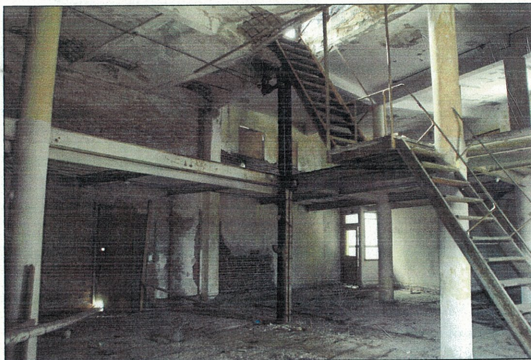
Photograph 22. Ferdinand's Building, interior, fifth floor.
