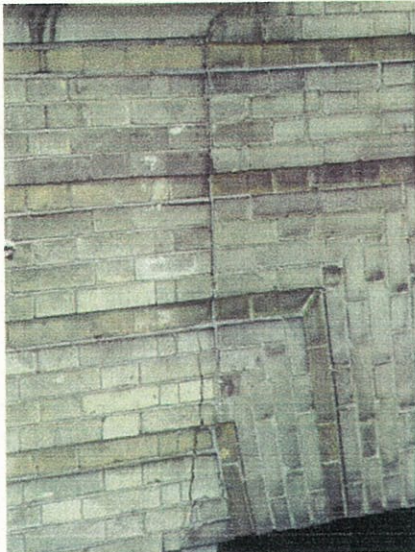
Photo 12: Joint between original building and addition at north elevation.
