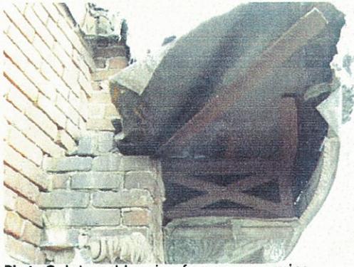
Photo 9: Internal bracing for copper cornice.
