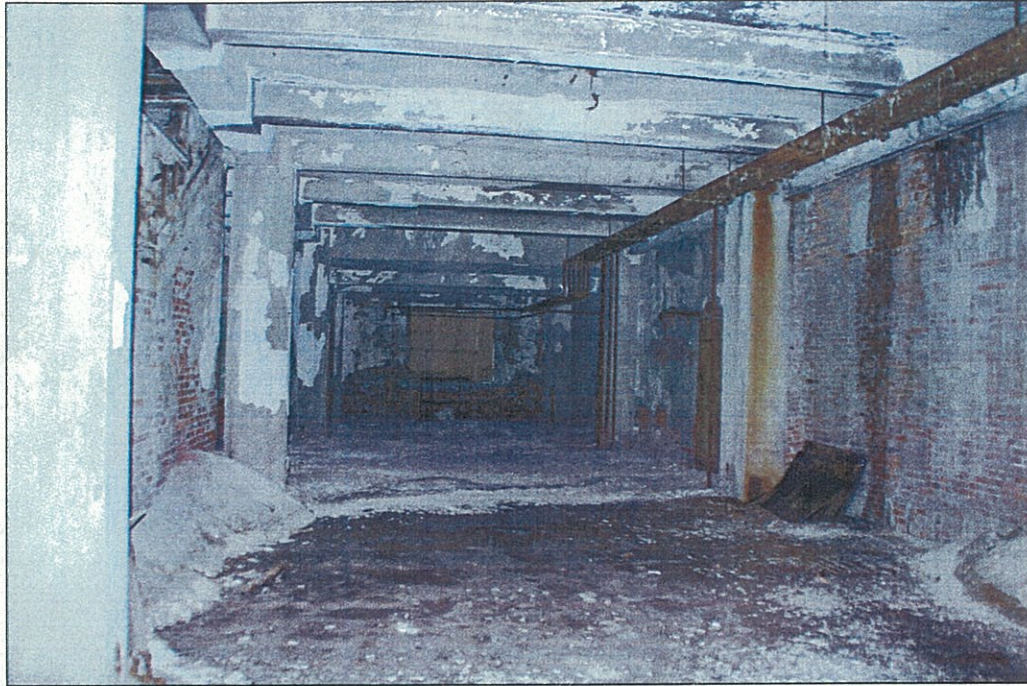
Photograph 13. Interior, basement typical view.
