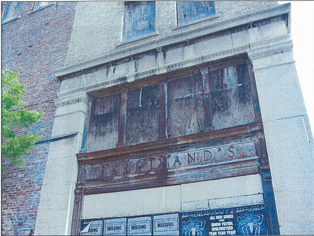
Photograph 9. Side elevation storefront detail, view north.
