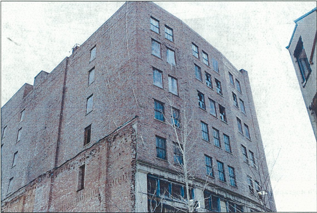
Photograph 4. Side and rear elevations, view southeast.
