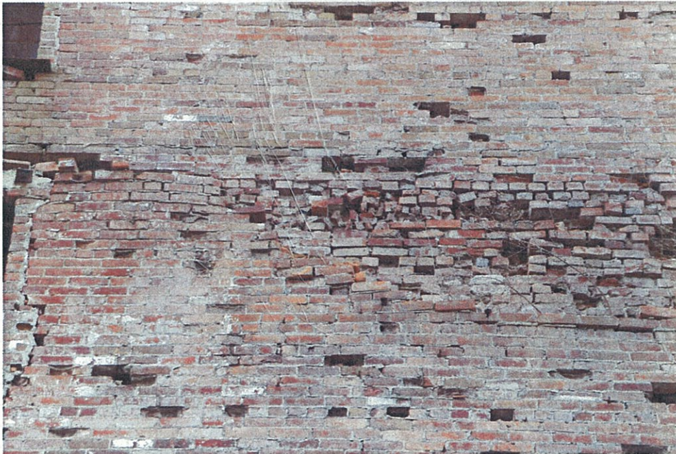
Photo GEX.4 – Exterior Wall
