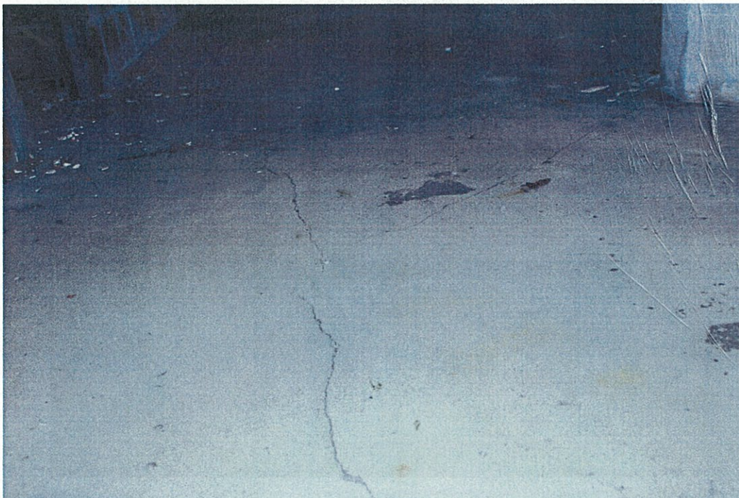
Photo G8.2 – 8 th Floor
