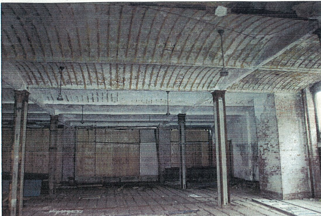
Photograph 21. Ferdinand's Building, interior, first floor.
