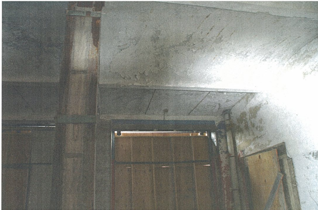
Photo F4.2 – 4 th Floor General interior elevation.
