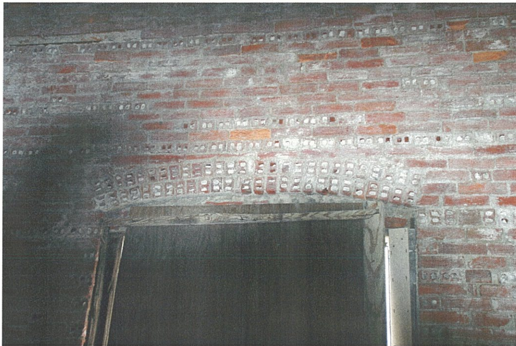
Photo F5.11 – 5 th Floor Masonry detail at a 5 th Floor window.
