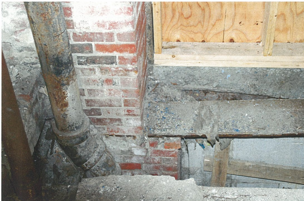
Photo F1.4 – 1 st Floor Looking down into opening in floor slab.
