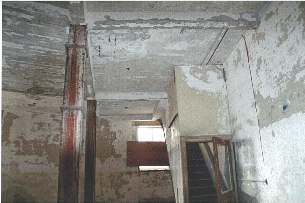
Photo F1.5 – 1 st Floor Stairway to 2 nd floor.
