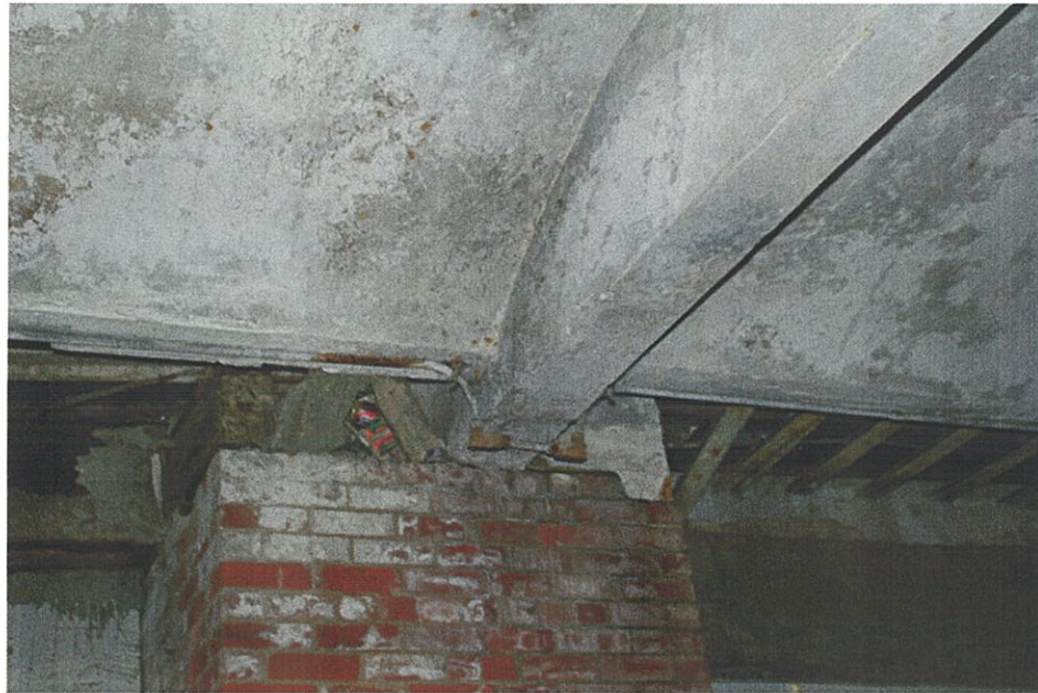
Photo F0.5 - Basement Connection of 1 st Floor framing to brick pilaster.
