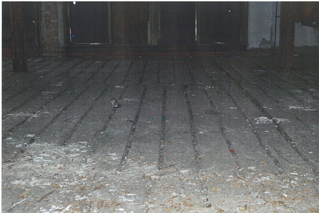
Photo F5.2 - 5 th Floor
