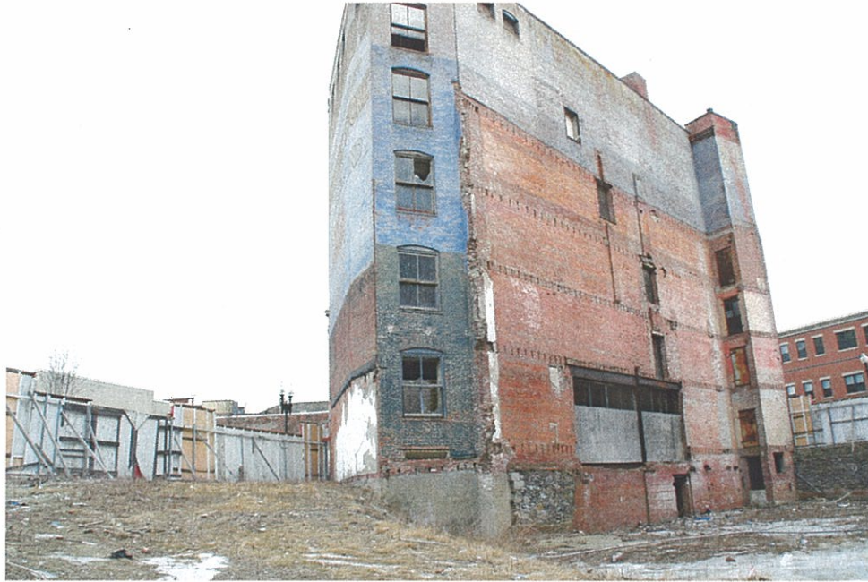
Photo FEX.4 – Building Exterior View from vacant lot.
