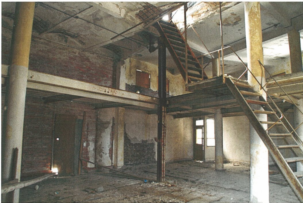
Photo F5.8 – 5 th Floor Stairs leading up to 5 th Floor mezzanine and to roof.
