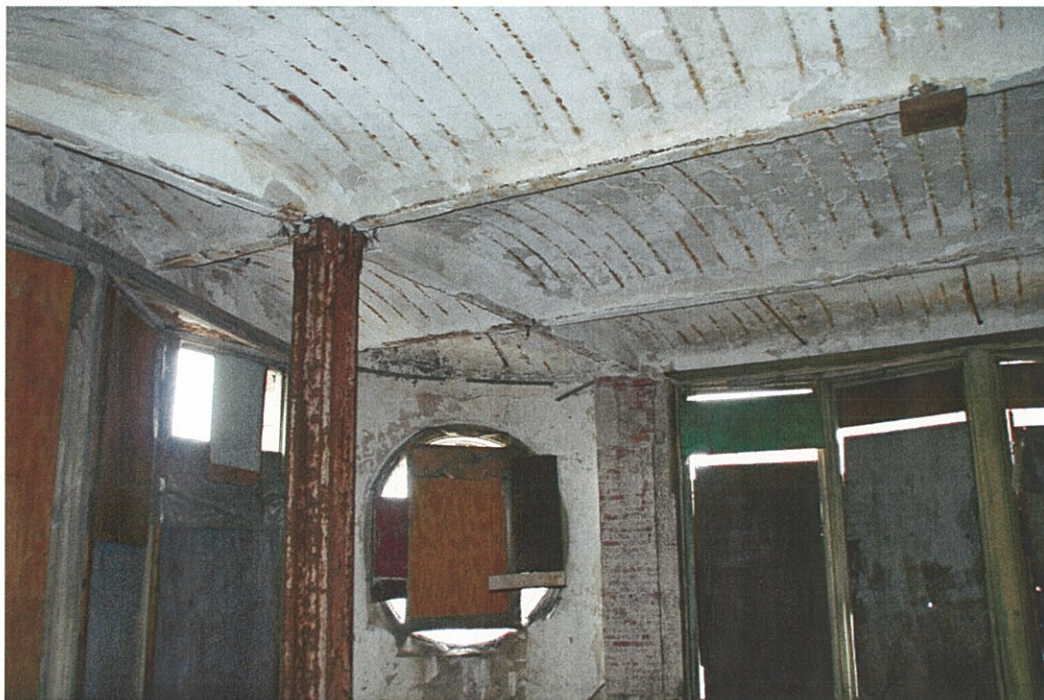
Photo F5.12 – 5 th Floor Elevation looking toward front ornate window.
