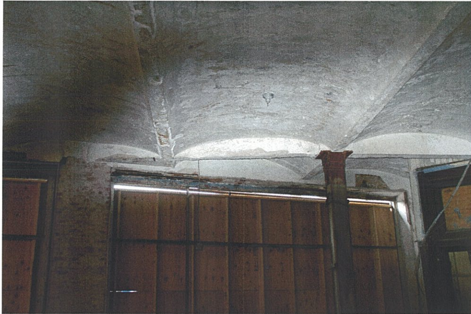
Photo F1.7 – 1 st Floor General interior elevation.
