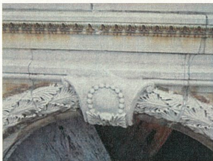
Figure 27. Portland cement repointing mortar in limestone joints.
