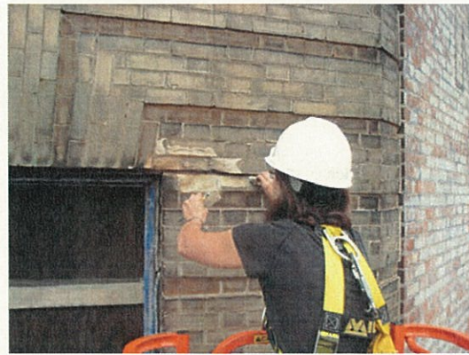
Figure 9. Removal of loose brick during survey.
