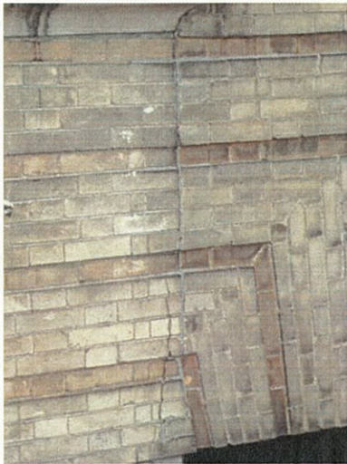
Figure 25. Joint between buildings.
