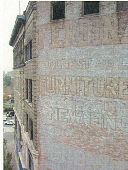
Figure 7. Full height painted wall sign.
