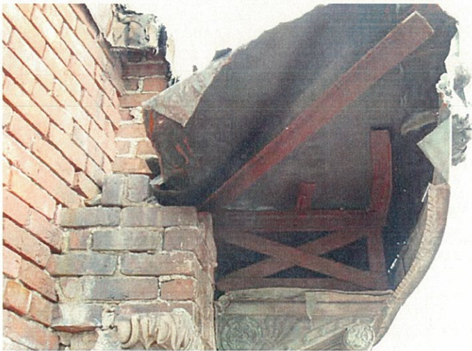
Figure 19. Interior bracing at cornice end (area of removal).
