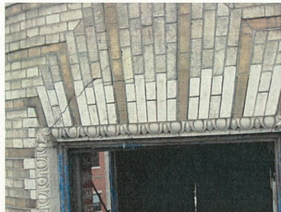
Figure 2. Three colors of brick around windows.
