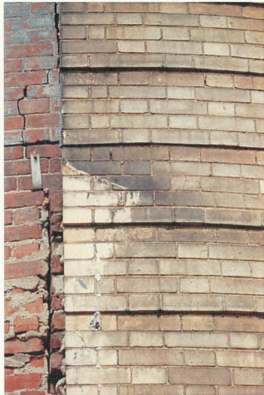
Figure 24. Joint between building and elevator shaft.
