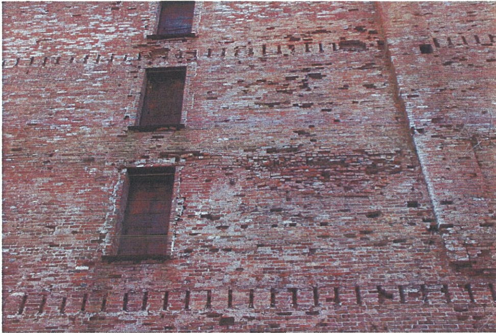
Photo GEX.3 – Exterior Wall
