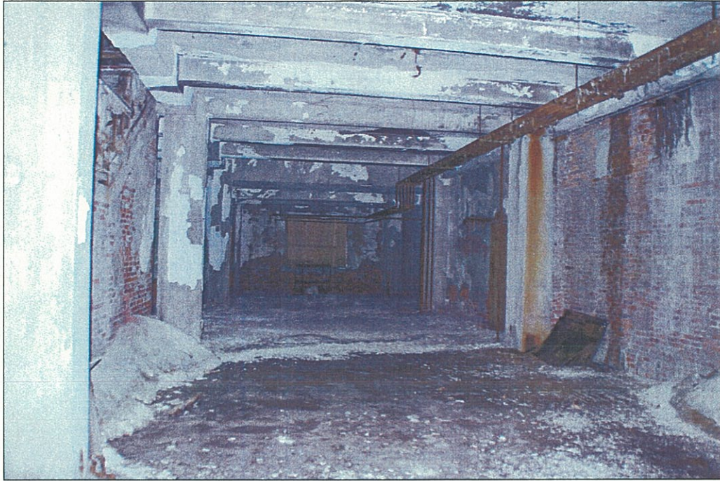
Photograph 13. Interior, basement typical view.
