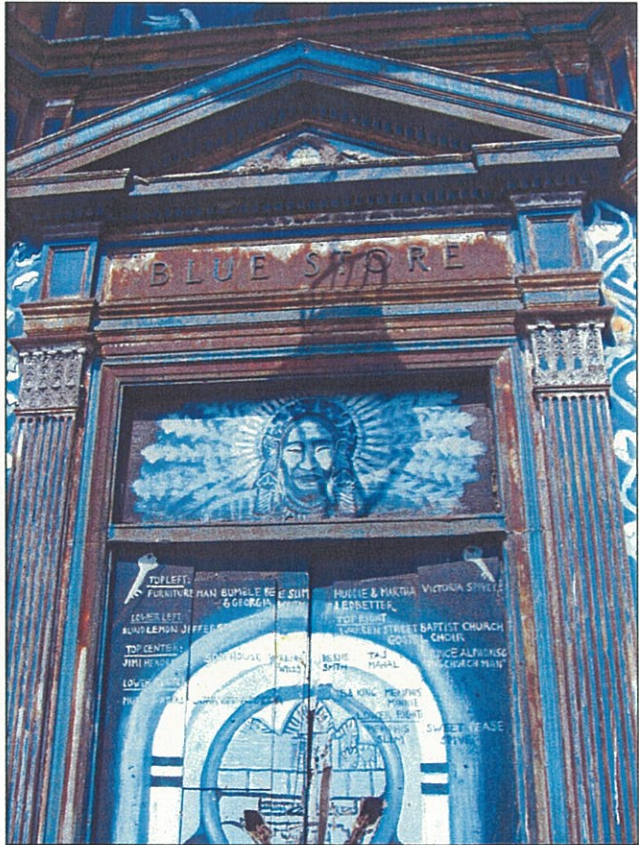
Photograph 10. Front elevation entrance detail, view west.
