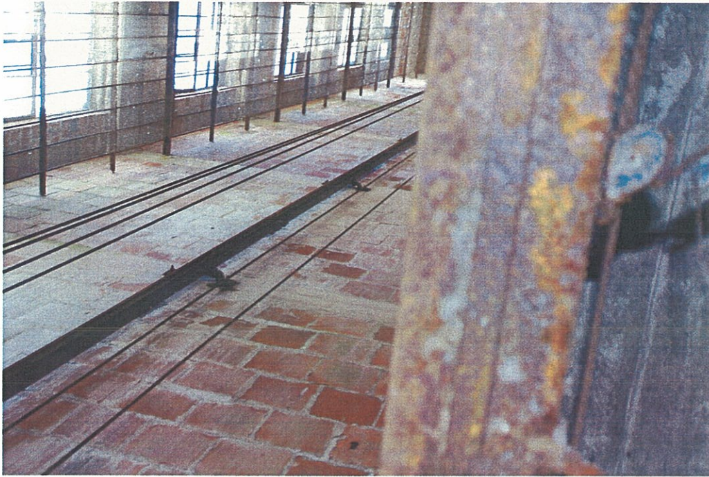
Photo G3.3 – 3 rd Floor
