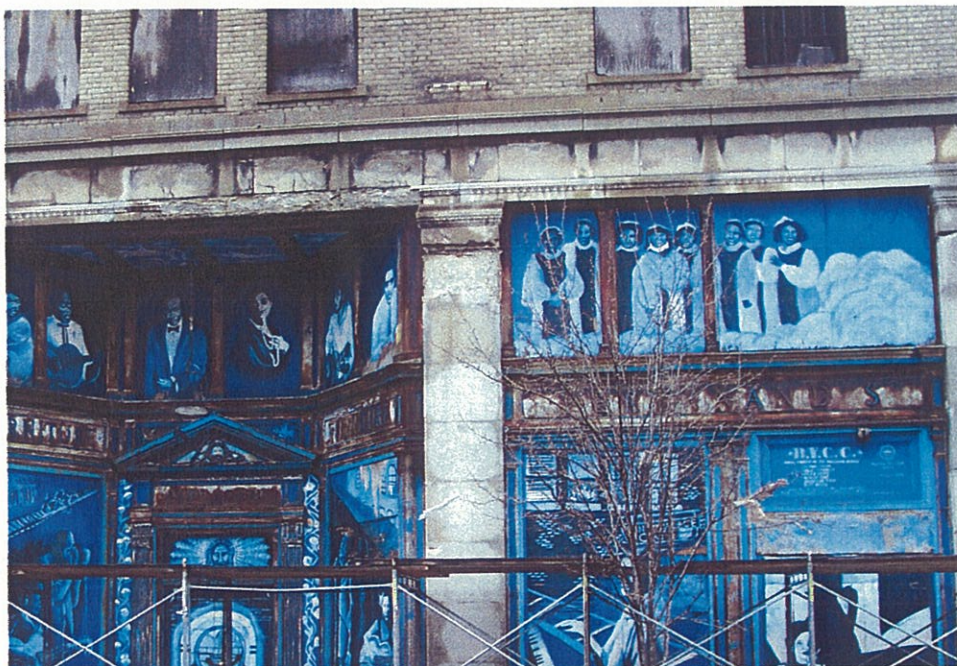
Photo GEX.8 – Front Entrance Scaffolding placed along sidewalk to protect pedestrians from falling debris.
