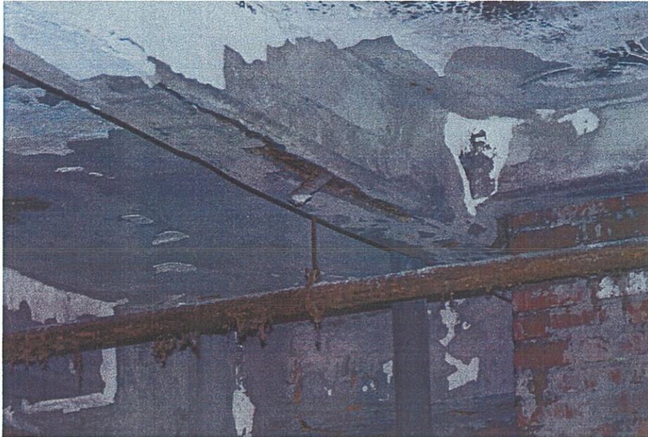
Photo G0.3 - Basement
