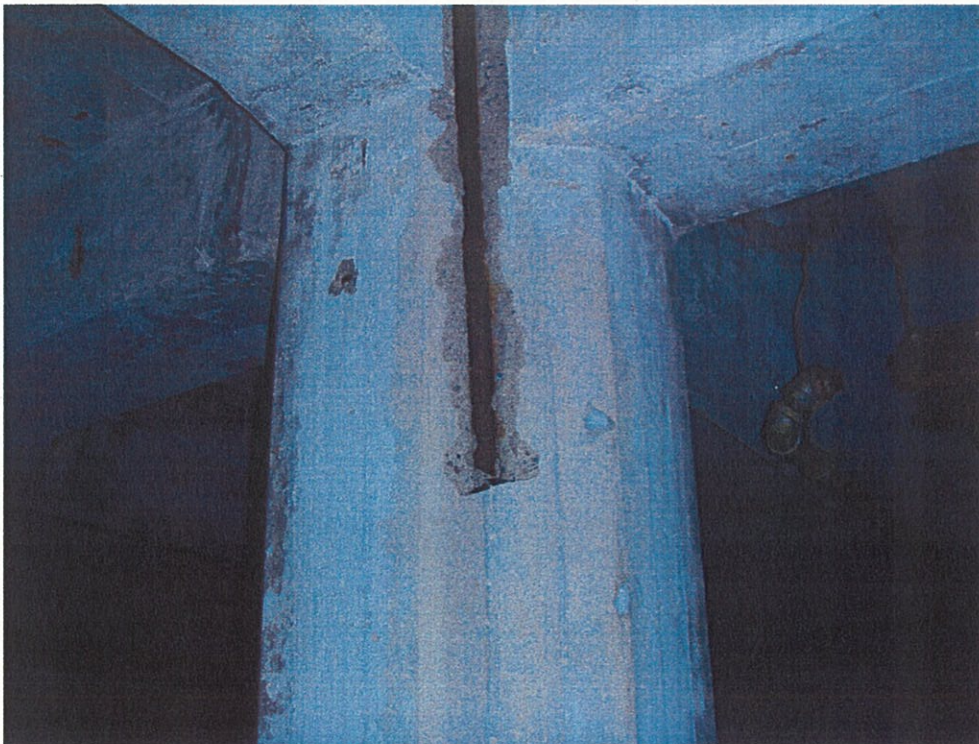
Photo CT0.4 – 4 th Floor Column Location of column where sample was taken.
