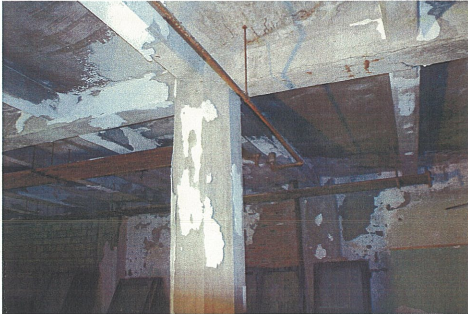
Photo G0.5 - Basement Typical beam-to-column framing.
