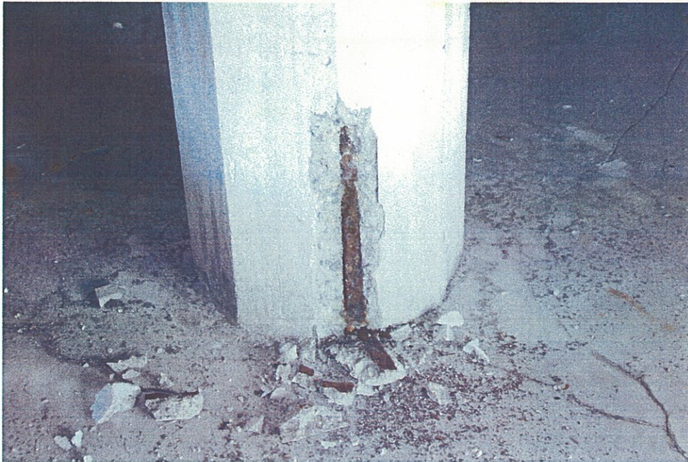
Photo G3.1 – 3 rd Floor
