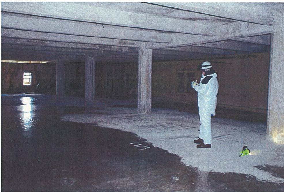
Photo G3.6 – 3 rd Floor
