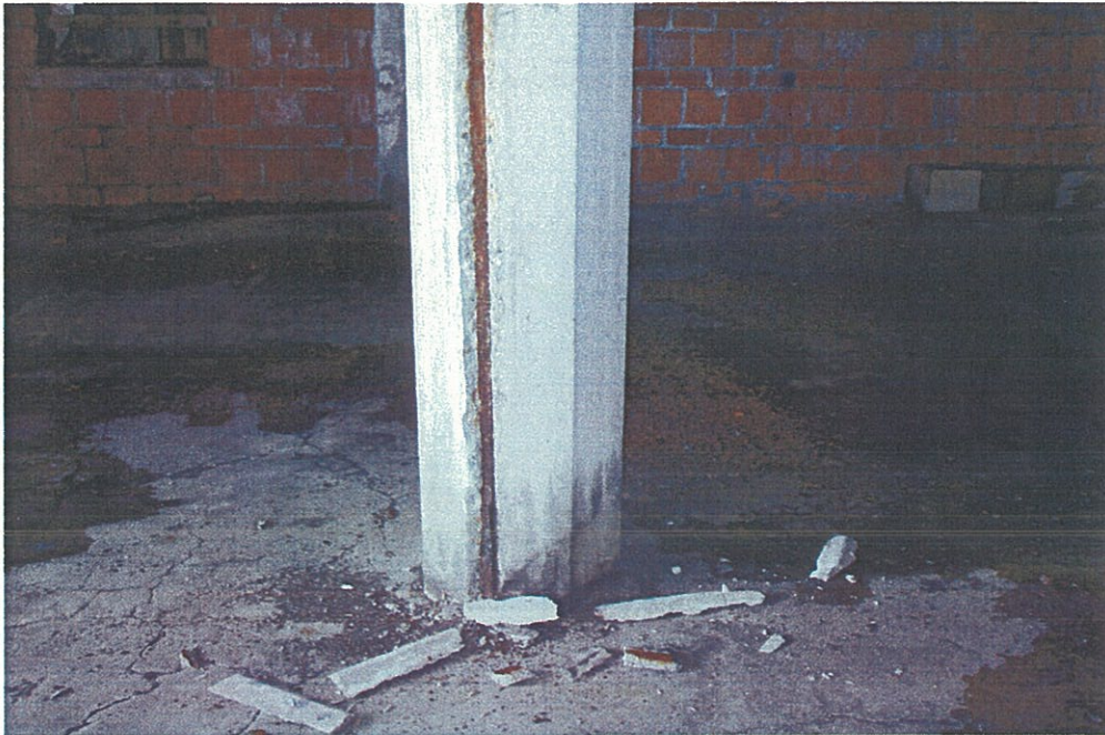
Photo G2.3 – 2 nd (Mezzanine) Floor
