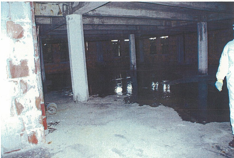
Photo G0.4 - Basement
