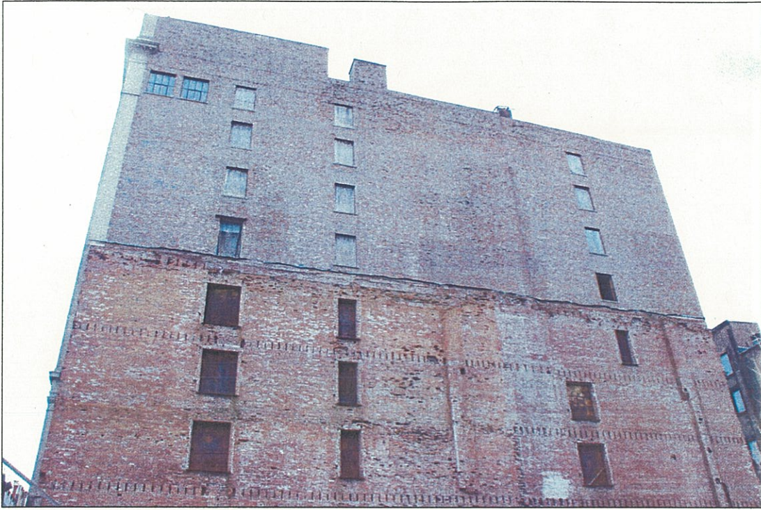
Photograph 5. Side elevation, view south.
