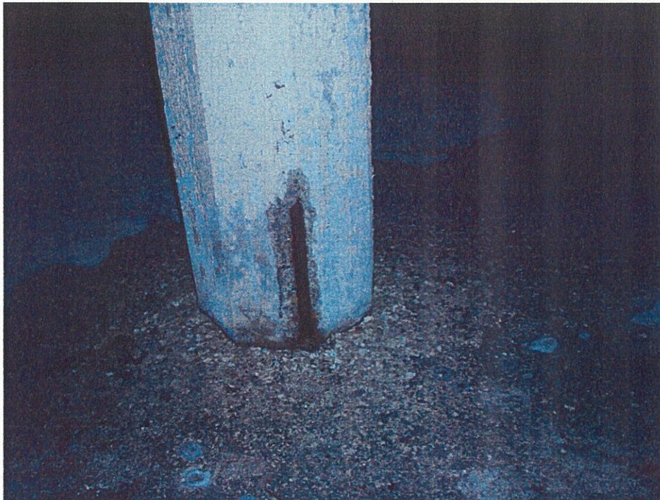
Photo CT0.6 – 5 th Floor Column Location of column where sample was taken.
