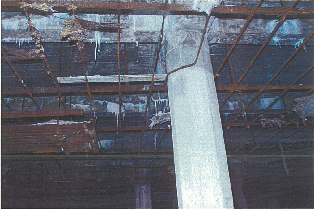
Photo G8.5 – 8 th Floor Ceiling framing suspended from structure above.
