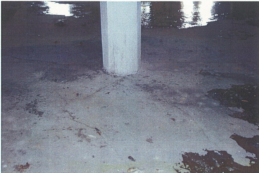
Photo G3.2 – 3 rd Floor
