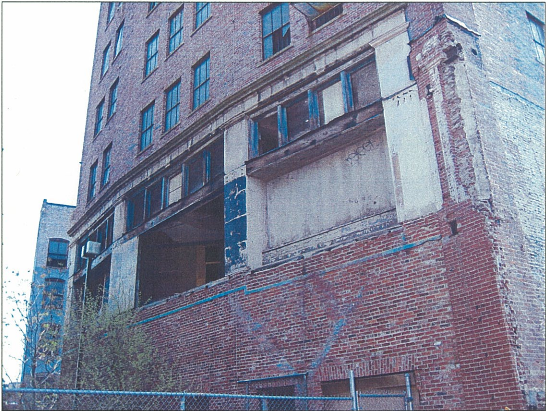
Photograph 8. Side and rear elevations detail, view northeast.
