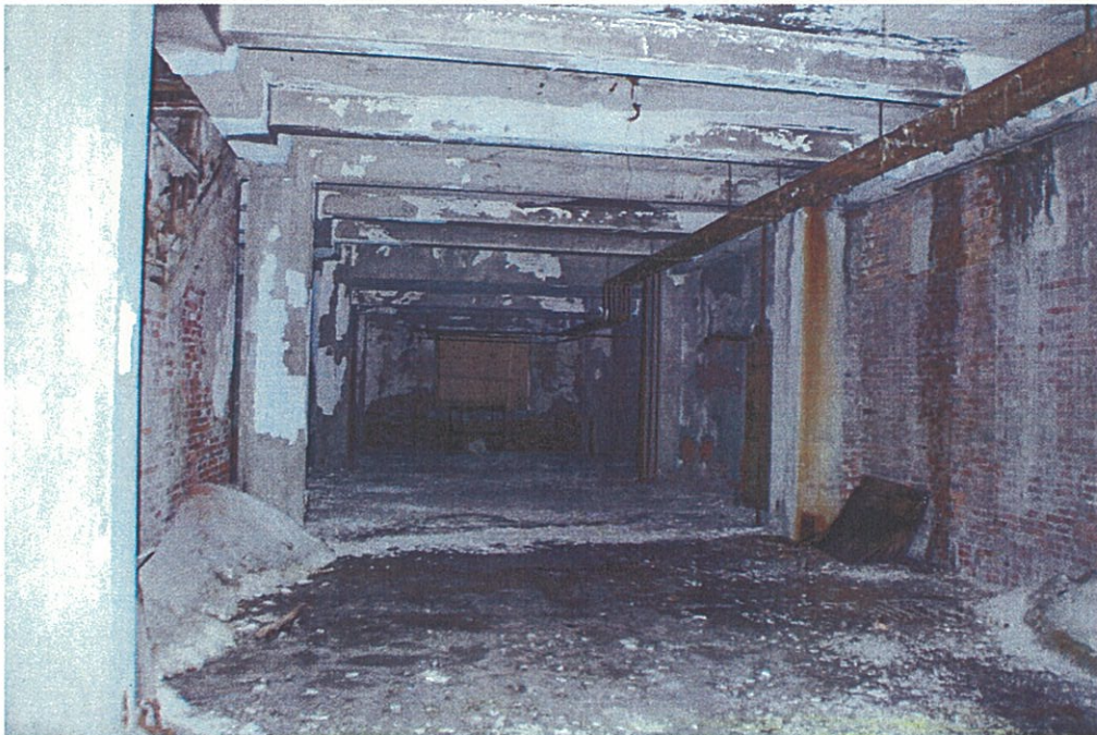
Photo G0.2 - Basement
