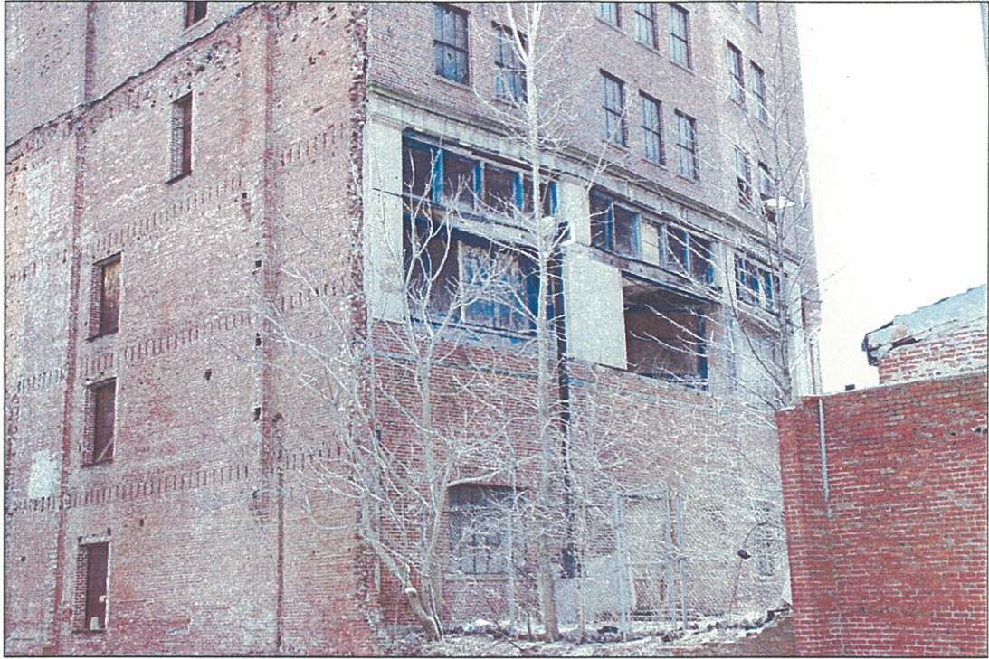
Photograph 7. Side and rear elevations detail, view southeast.
