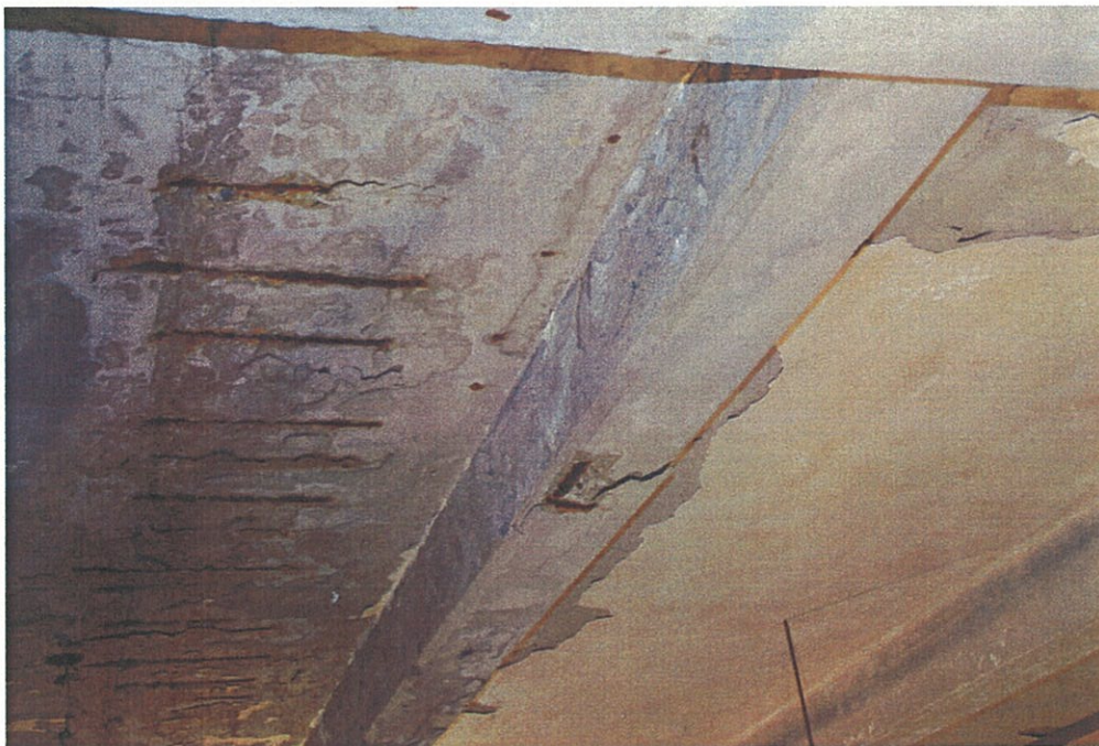
Photo G2.4 – 2 nd (Mezzanine) Floor
