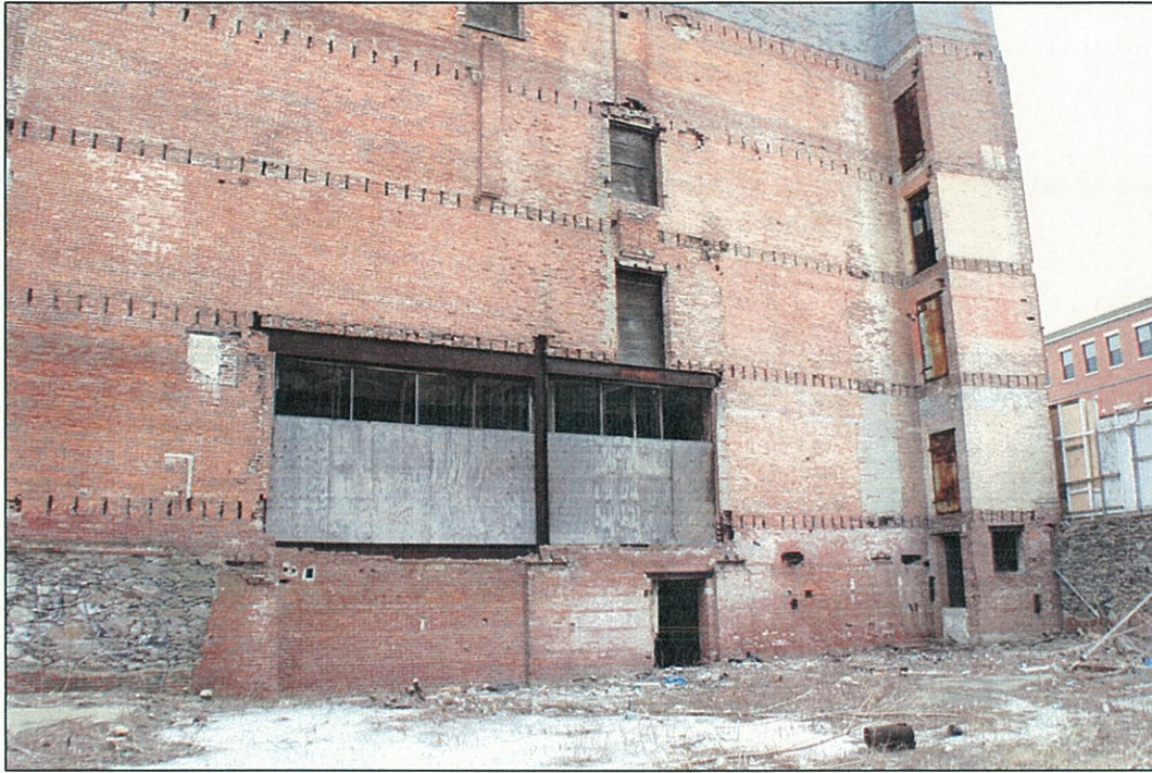
Photograph 7. Ferdinand Building rear elevation and shaft, view north.
