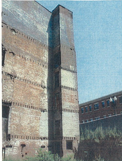
Figure 1: Ferdinand Building - Warren Street Elevator Shaft Elevation view as seen from vacant lot
