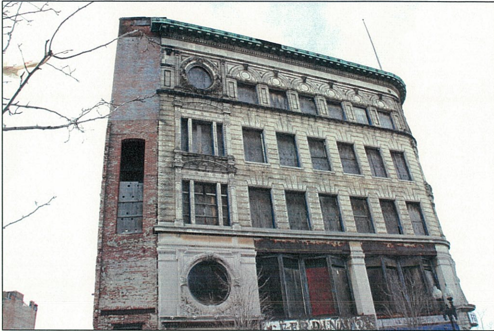
Photograph 5. Ferdinand Building façade, showing elevator shaft, view west.
