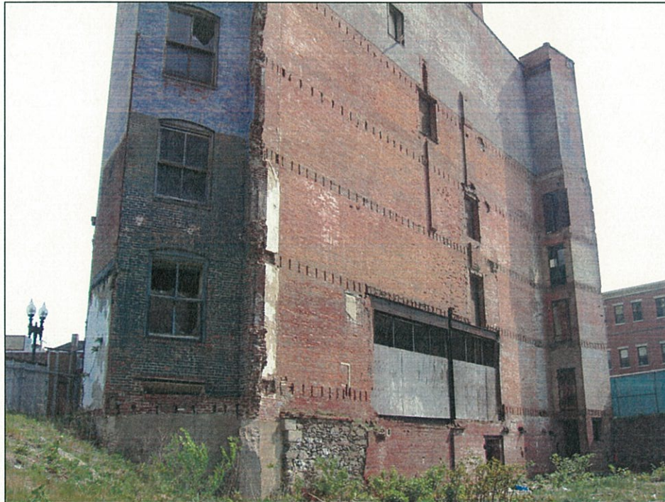
Photograph 4. Ferdinand Building side and rear elevations, showing elevator shaft, view northeast.
