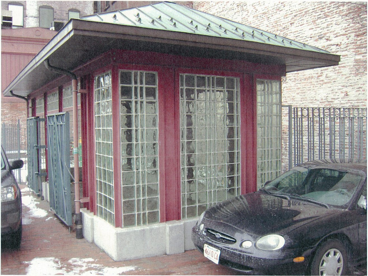
Photograph 8 MBTA Bus Shelter
