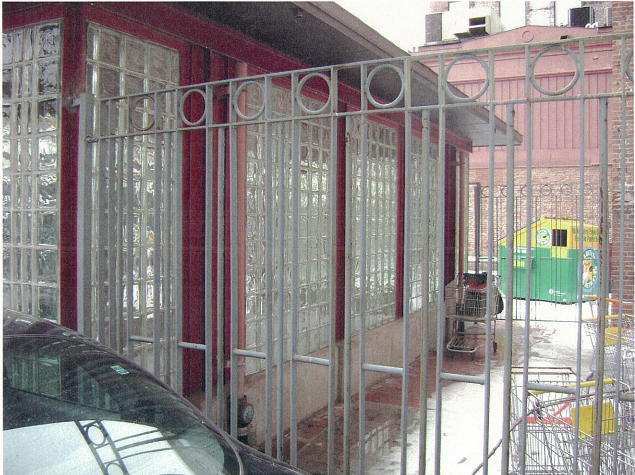
Photograph 9 MBTA Bus Shelter
