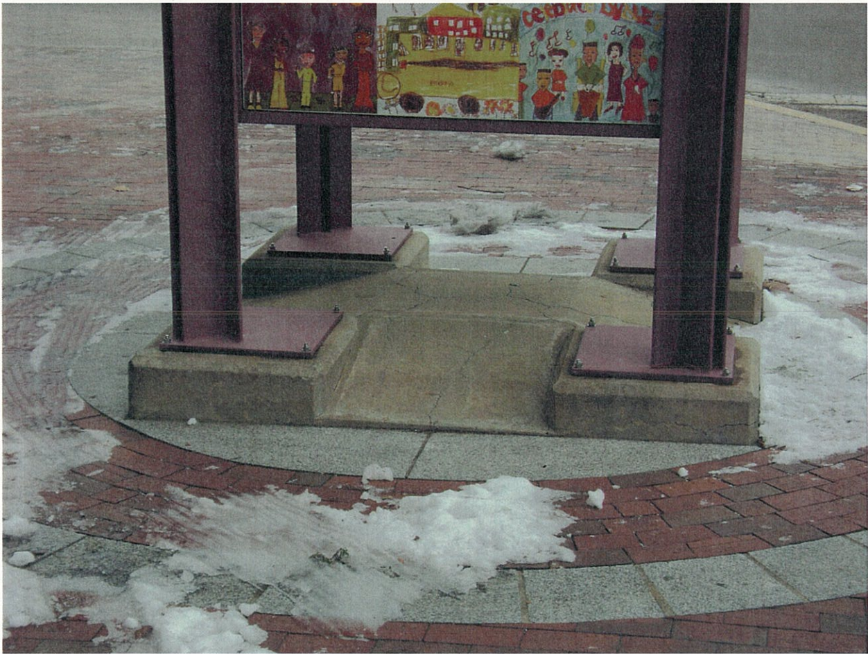
Photograph 11 MBTA Sign Base
