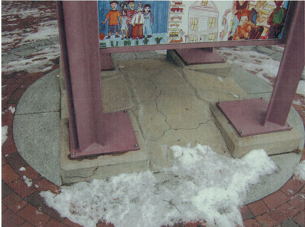
Photograph 12 MBTA Sign Base
