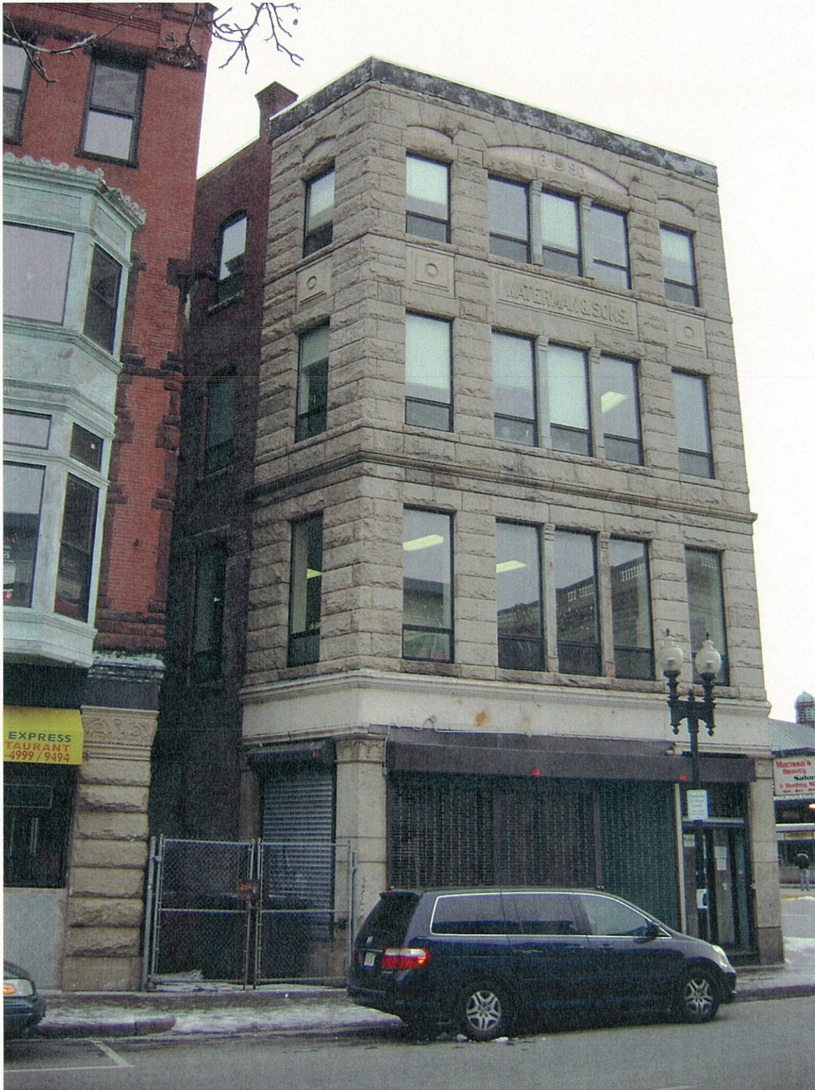
Photograph 26 No. 2328 Washington St. West Face
