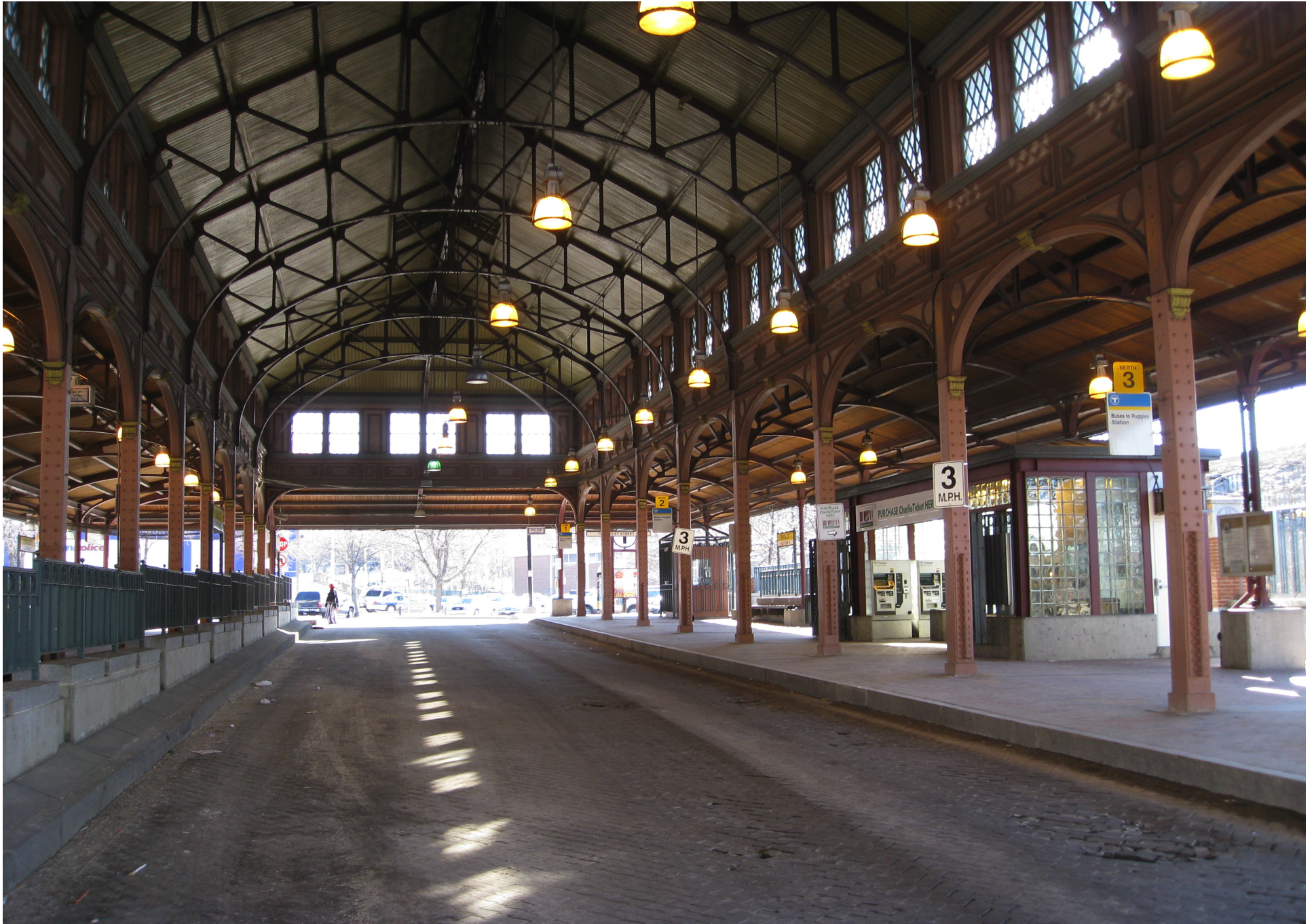
View of Interior of Dudley Square Station
