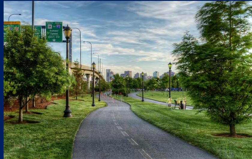
12 foot-wide bituminous concrete paved multiuse trail.
