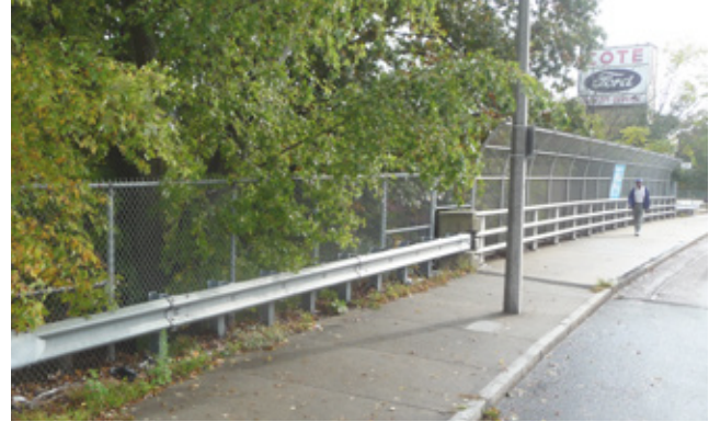
The location of the station entry on Cummins Highway is separated from the activity of Mattapan Square
