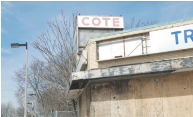
Focusing transit-oriented housing near the train station takes advantage of the location
