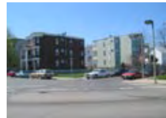
The majority of the housing in the CSNDC area is comprised of triple-deckers.
