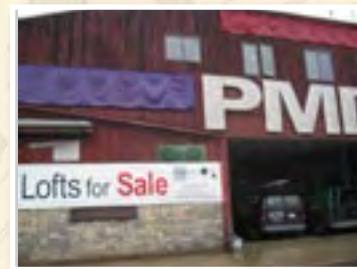
An abandoned lumber yard was recently converted into artists' live/work homeownership units. This development located between the Fairmount and Readville stations straddles the Neponset River.
