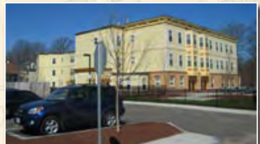
The Talbot-Bernard village community developed by CSNDC added 75 family and senior units on a brownfield site.
