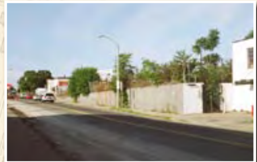
A vacant parcel along Hyde Park Avenue near the Readville Station needs redevelopment.
