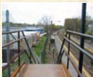
The Morton Street station requires stairways from a bridge over the tracks.
