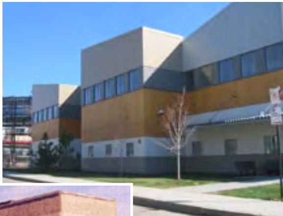
The Spire building brought 140 jobs onto a former brownfield site and won the EPA's "Phoenix Award."
