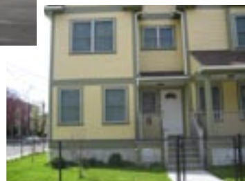
MCDC developed these affordable and energy efficient units on a street of triple-deckers.
