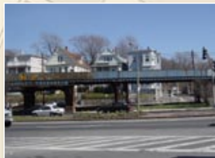
East of Columbia Road the new station would serve nearby Bowdoin Street neighborhoods.
