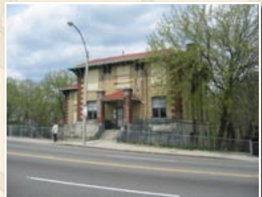
A historic police station building sits immediately north of the station and slated for redevelopment as housing.
