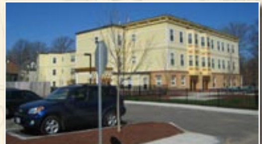
The Talbot-Bernard village community developed by CSNDC added 75 family and senior units on a brownfield site.
