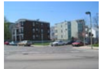
The majority of the housing in the CSNDC area is comprised of triple-deckers.
