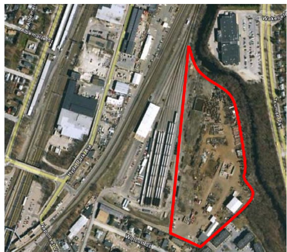
Figure 4.1: Potential Site of New Maintenance and Storage Facilities Next To Readville Yard
