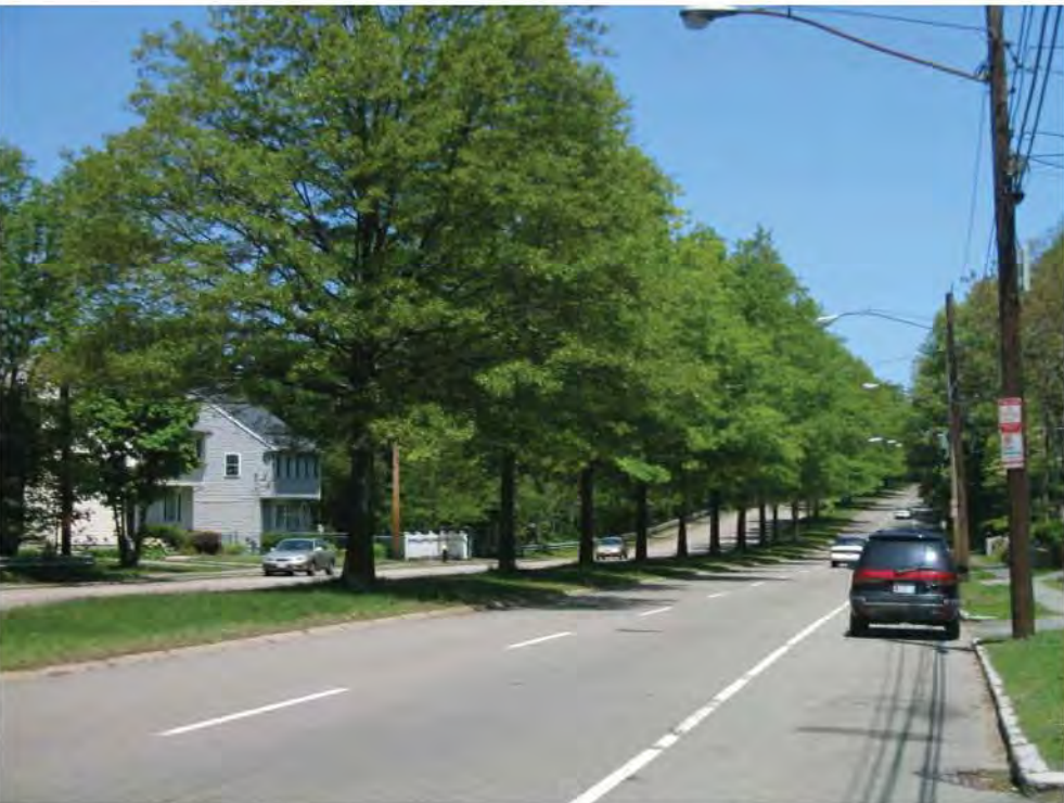
Truman Parkway Looking North
