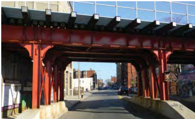
The rail overpass at Upham’s Corner Station
