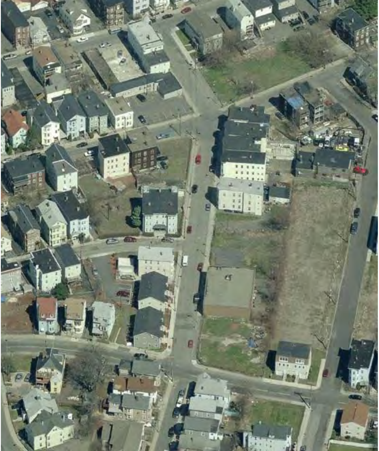
The aerial image (below) shows the type and scale of infill redevelopment opportunities in the residential neighborhoods surrounding Upham's Corner
