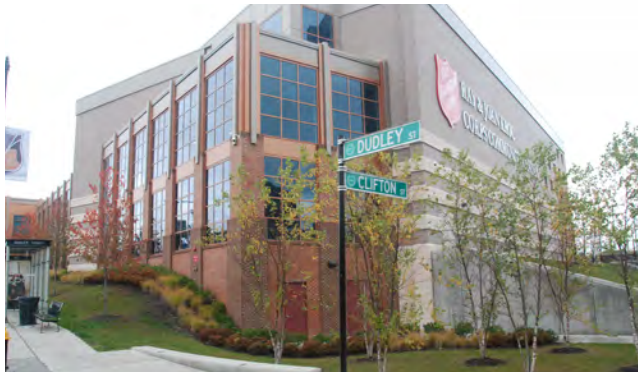
The Salvation Army's Kroc Community Center
