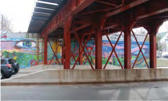
Overpass at the rail station entry on Dudley Street
