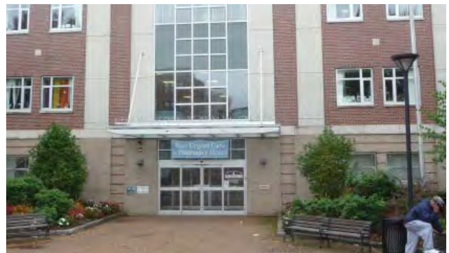
Upham's Corner Health Center
