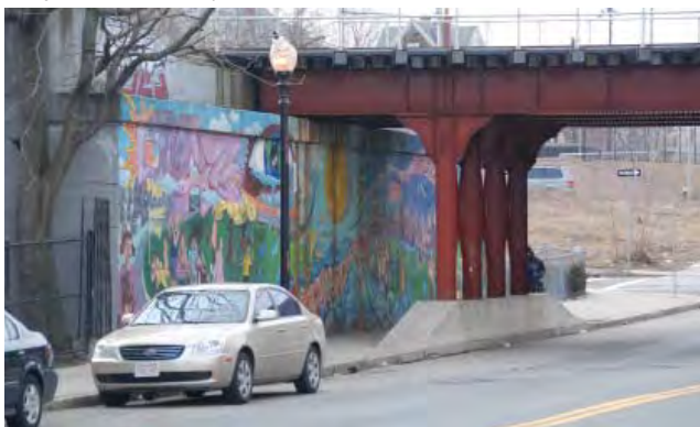
A bridge overpass above Dudley Street at the Rail Station
