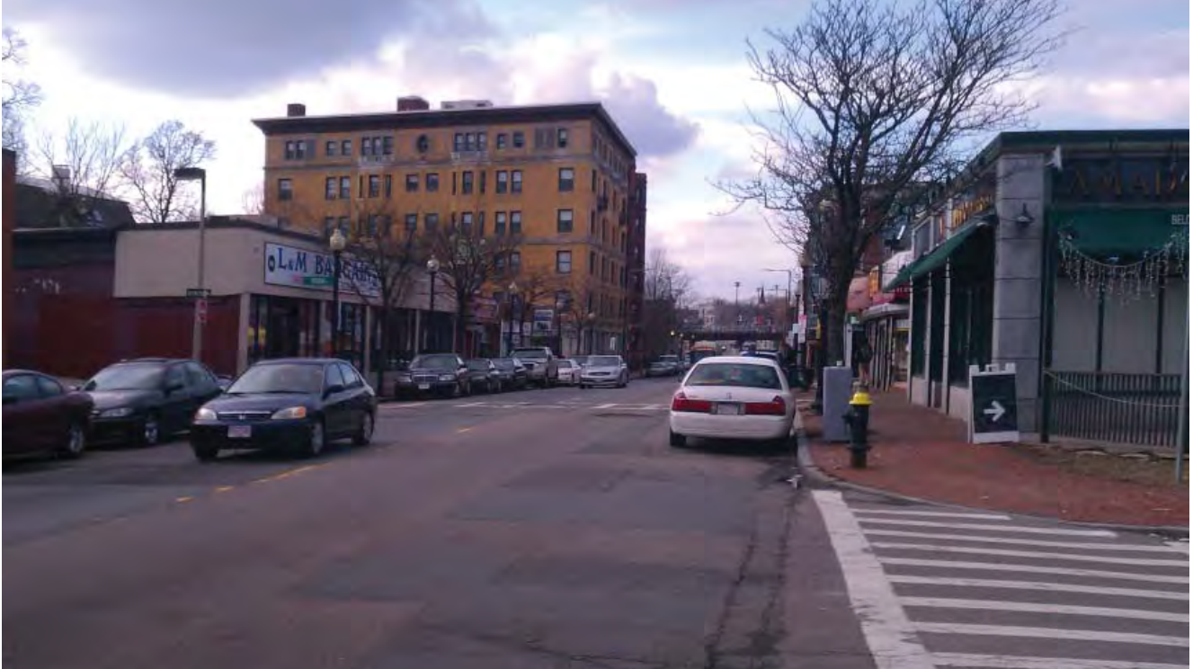
Dudley Street Existing Conditions
