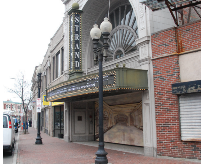
The Strand Theatre a cultural anchor to Upham's Corner
