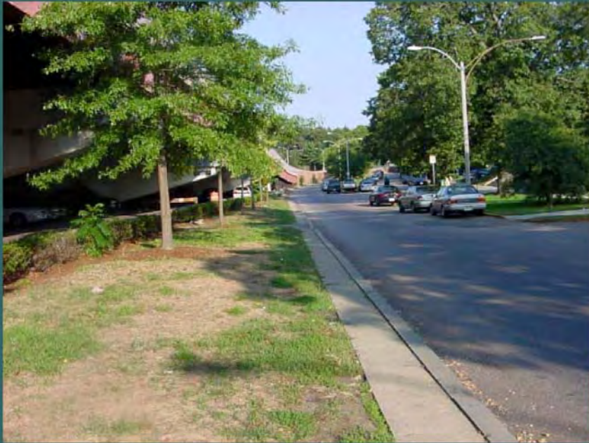
Under Casey Overpass - Existing
