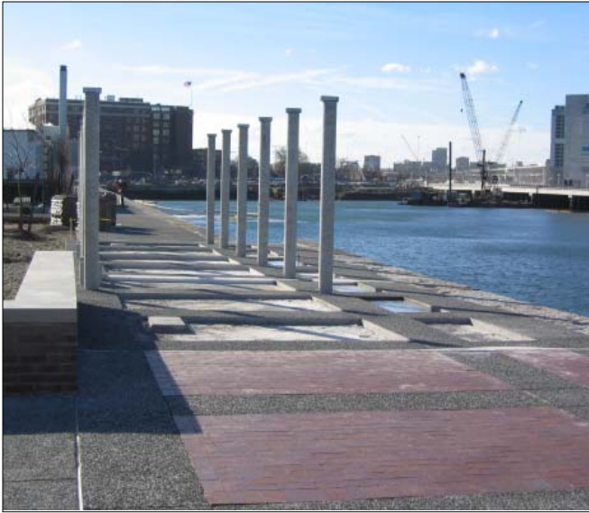
Harborwalk under construction along Gillette property, 2004
