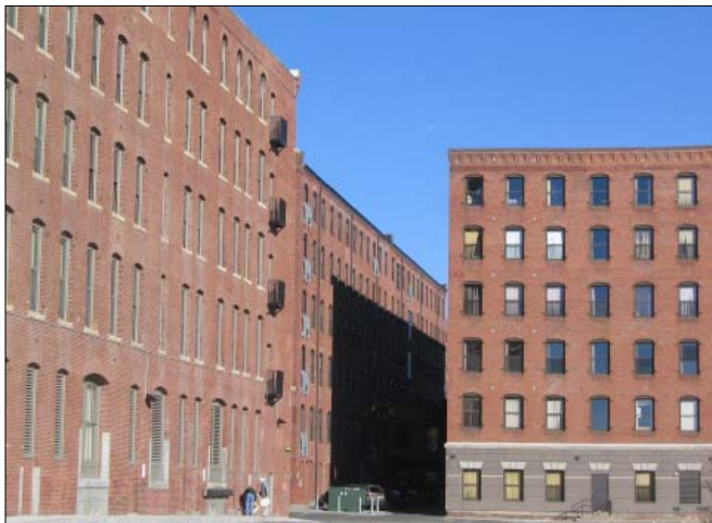
Existing Wharf Buildings
