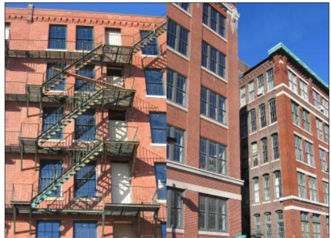
Existing Architectural Features
