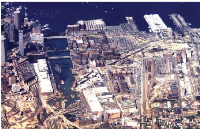
Central Artery Tunnel Project Construction in South Boston
