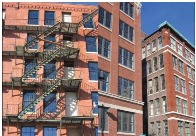
Existing Architectural Features
