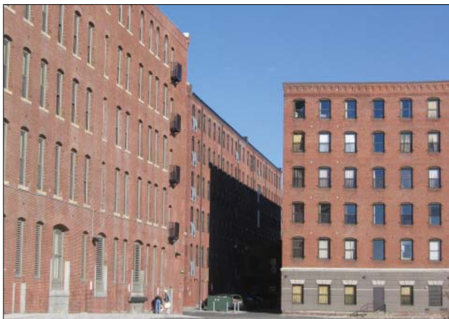
Existing Wharf Buildings
