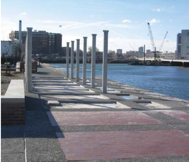
Harborwalk under construction along Gillette property, 2004
