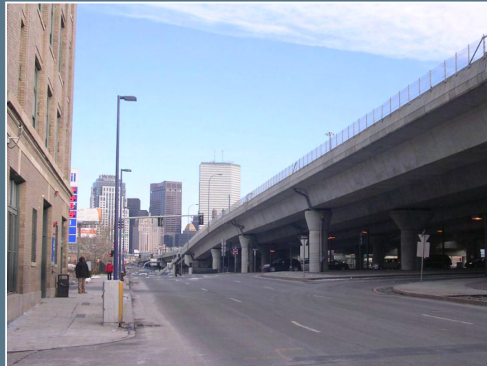
Elevated Highway & Viaducts
