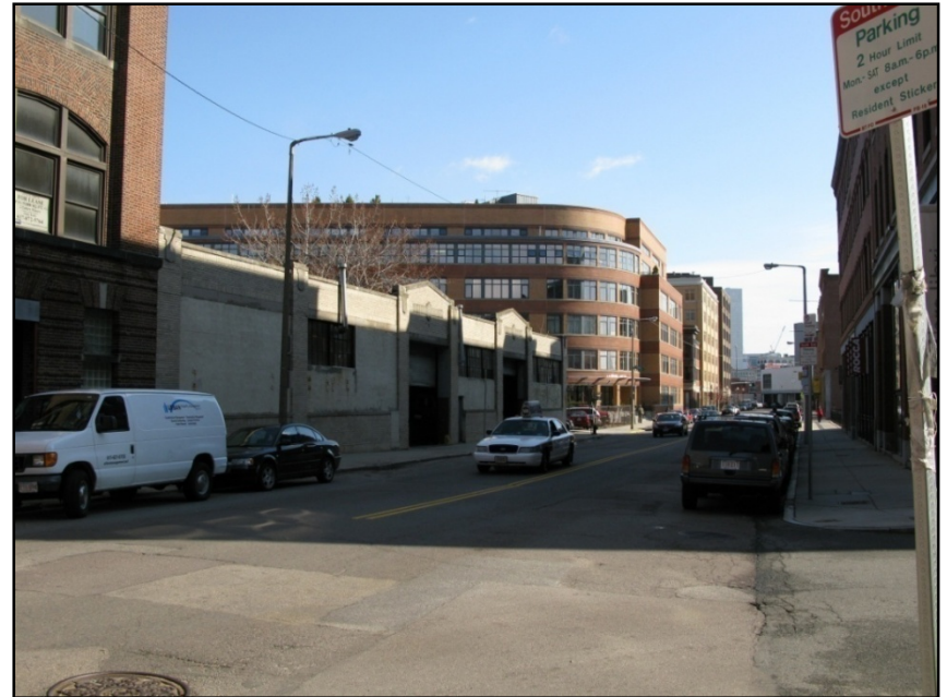
Land Value Potentially Exceeds Building Value ?
