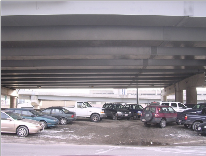
Surface Parking Under Expressway Viaducts
