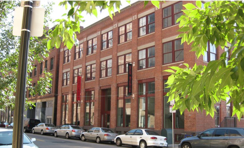
Converted industrial building on Harrison Avenue
