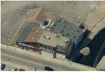
The PMDI Building on Hyde Park Avenue is an example of artist live-work space.
