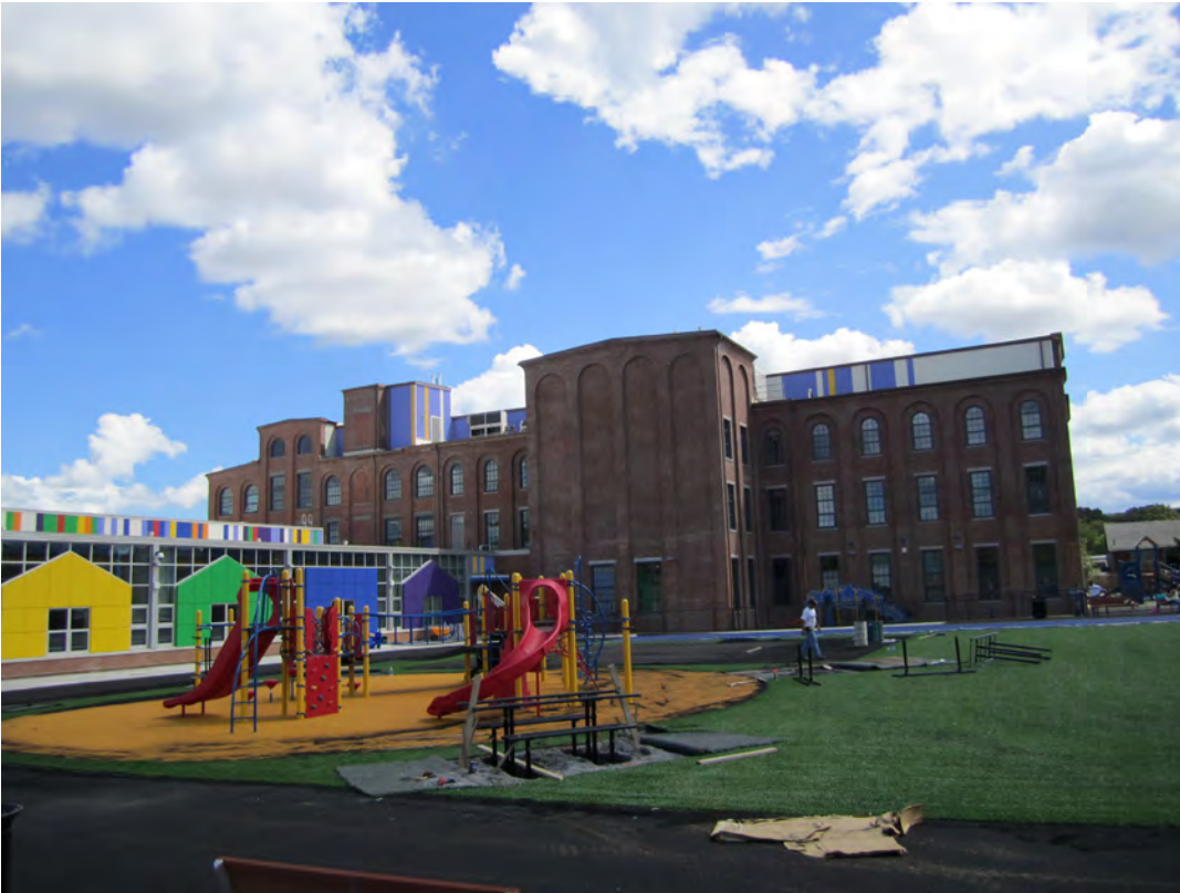
The newly opened Renaissance charter School in the former American Tool and Machine Company Building, is a beautiful example of an adaptive reuse of an historic building.
