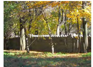
The alignment along Edgewater Street would require breaching this historic stone wall.
