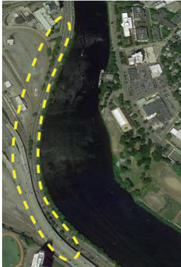
Existing Conditions, Soldiers Field Road and Charles River Edge
