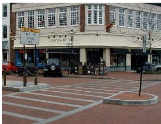
Intersection with a median nose and opening the full width of the crosswalk.
