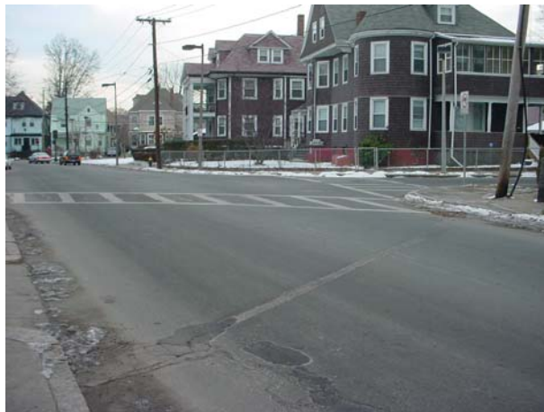
Amory Street looking north towards School Street and Marbury Terrace. Note faded double yellow line. The recently marked diagonal crosswalk lengthens the crossing distance. There are no wheelchair ramps.
