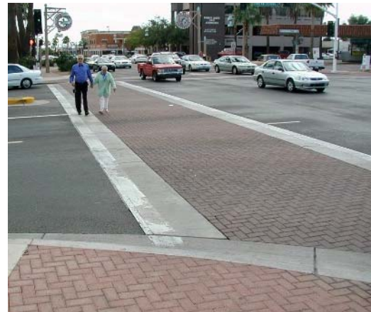
Distinctive paving material can make crosswalks more visible and attractive.
