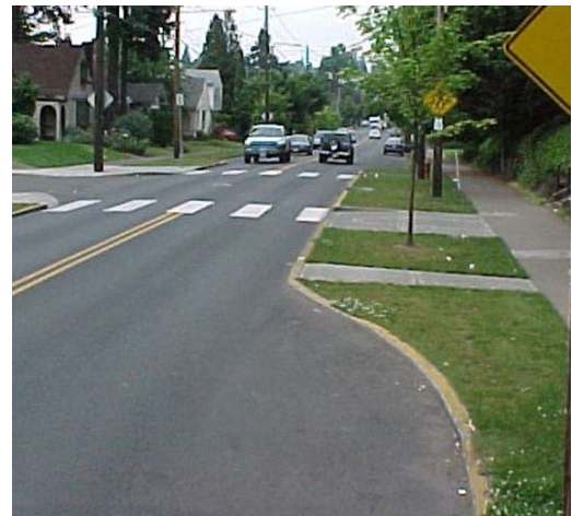
Curb extension with trees and landscaping.
