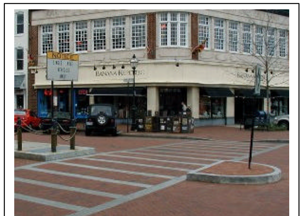
Intersection with a median nose and opening the full width of the crosswalk.
