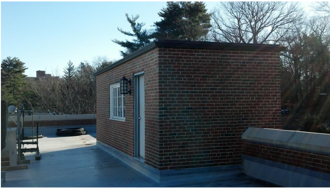
Existing Building Roof
