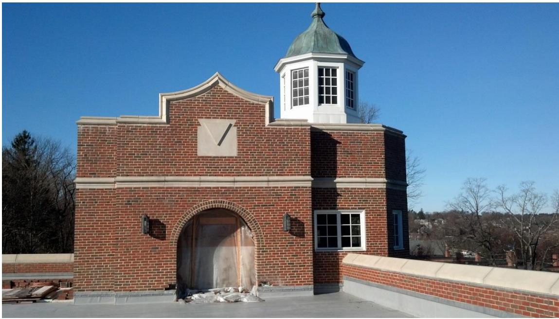
Existing Building Roof
