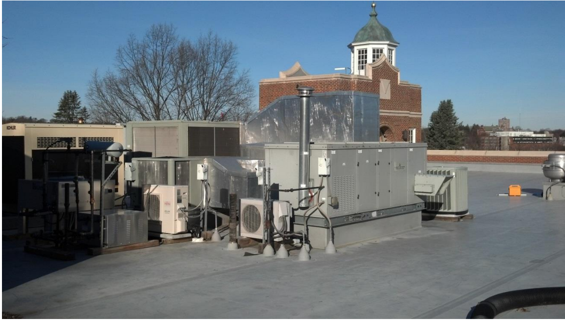
Existing Building Roof
