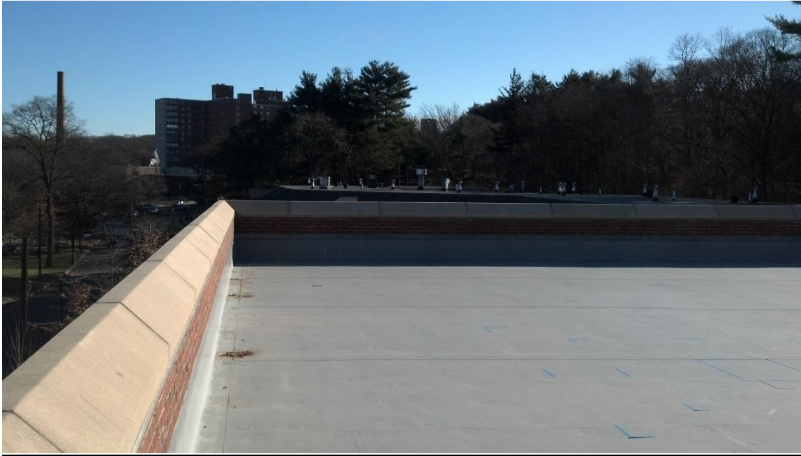
Existing Building Roof
