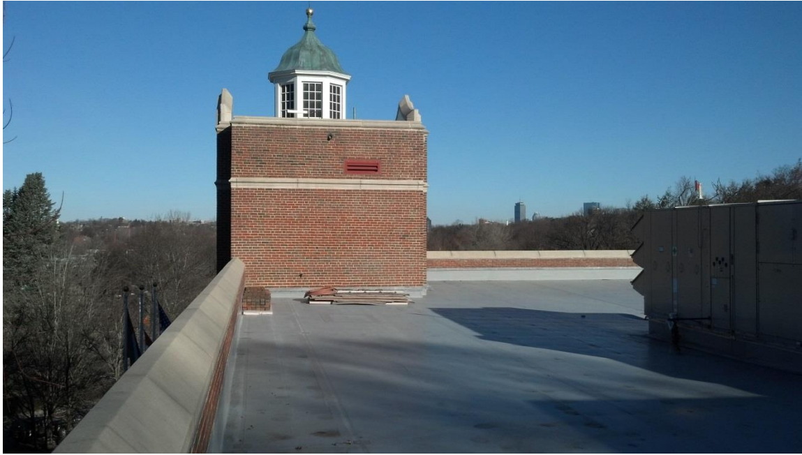
Existing Building Roof
