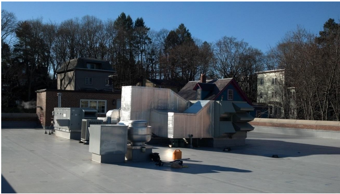
Existing Building Roof
