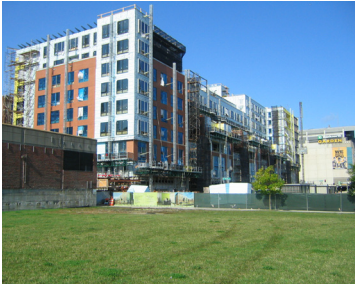
Avenir under construction
