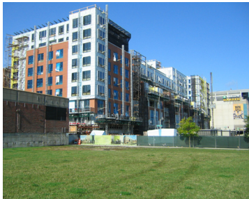
Avenir under construction
