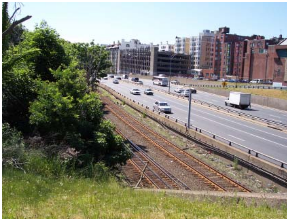
Parcel 12 - Looking Northwest
