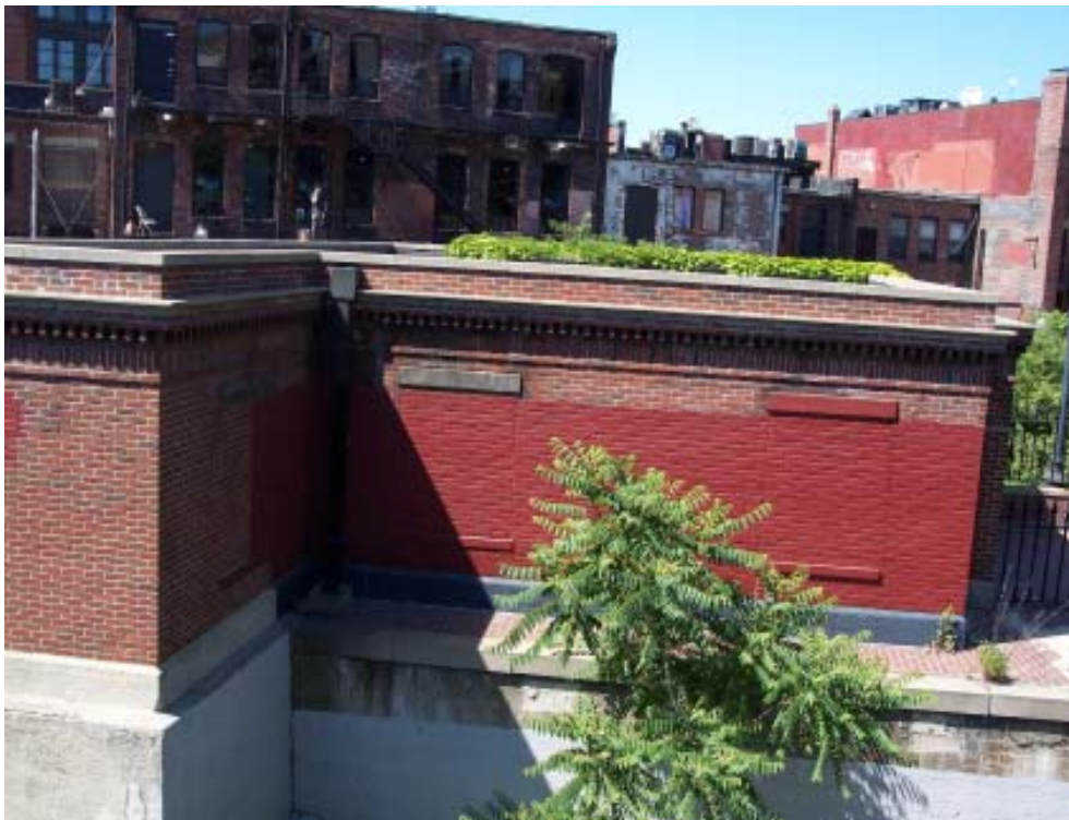
Parcel 13 - MBTA Station Exit
