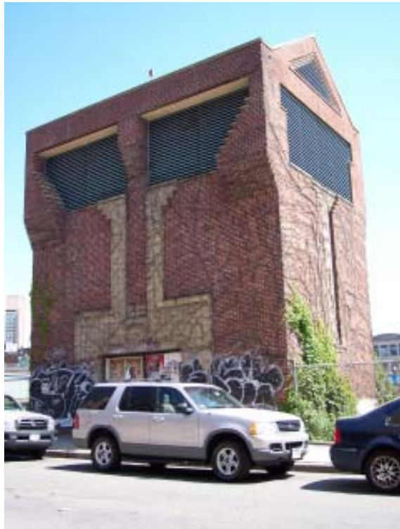
MBTA Vent Building at Parcel 12
