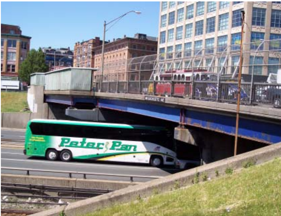
Parcel 12 - Looking Northeast
