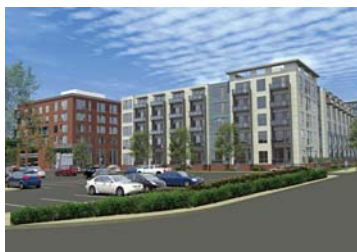
Morrissey Boulevard Residences
