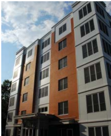
Franklin Hill Redevelopment
