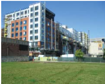
Avenir under construction
