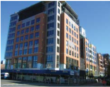
Avenir under construction
