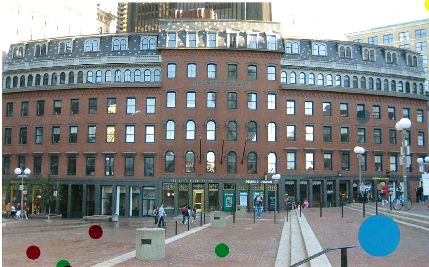
Sears Crescent Building, Government Center
