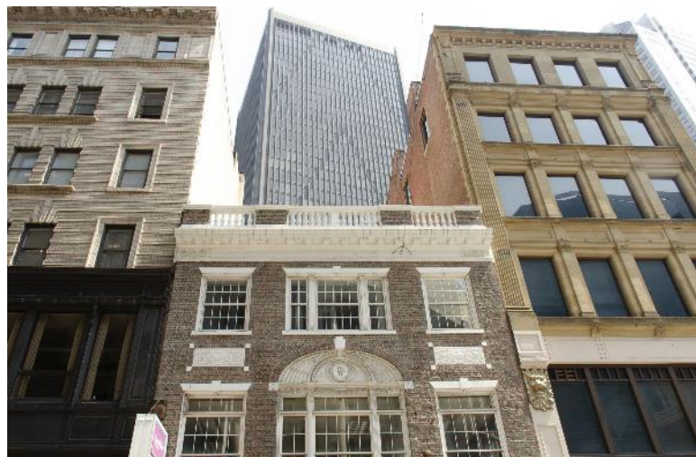
21 School Street, Downtown Crossing
