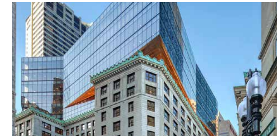
The Congress Square project by Arrowstreet in 2015 adaptively reused existing historic buildings, restored existing facades, and added a modern addition above the existing historic structures.
