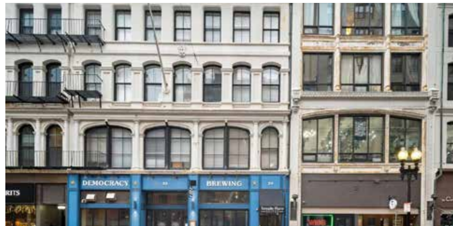
Historic facades of 37 Temple Street
