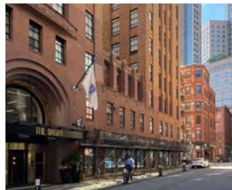
Relationship of the Batterymarch Building facade (1918) to the frontage of Broad Street
