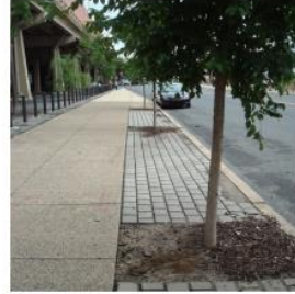
Stormwater Tree Trench
