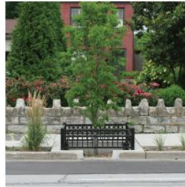
Stormwater Tree Pit
