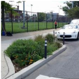
Stormwater ROW Bumpout
