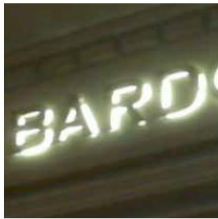
Halo Illumination Projected light from behind individual letters or symbols gives a halo effect.
