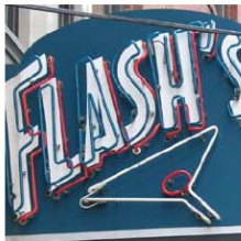
Exposed Neon Tube Light is emitted by neon tubes mounted directly to the face of a sign.
